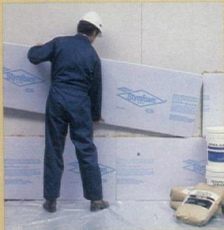
Boards of STYROFOAM brand insulation are set in place
