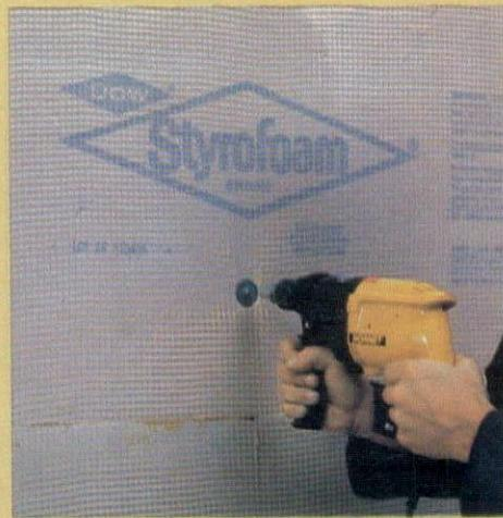
Fiberglass mesh is applied, mechanical anchors are attached
