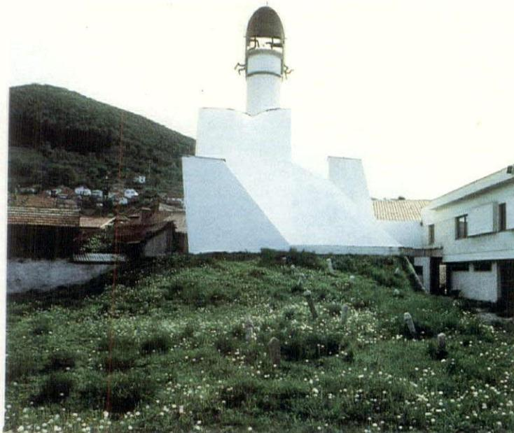
*The new mosque, while somewhat larger than Visoko's principal mosque which it replaces, remains in good scale with its surroundings, yet stands out from them as an important landmark. The entire building is of reinforced concrete. Its exterior is surfaced with stucco painted white and the interior walls are covered with white mortar. The sinuous green-painted iron tube that wraps the top of the minaret recalls Kufic calligraphy and also serves as an illuminating device.*
