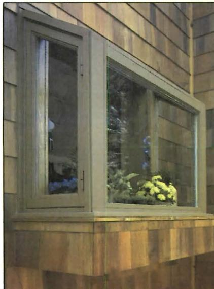
of fine-grained Ponderosa pine. This wood was chosen for its excellent insulating properties and the way it accepts a stain-and-varnish, or paint, finish.
