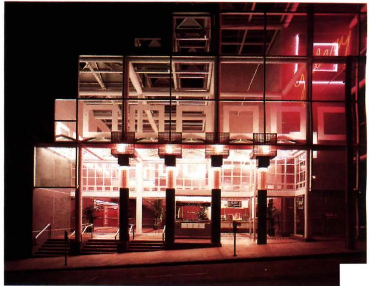
*At the Galaxy Theaters, green-tinted glass rises in steps to the topmost cube 75 feet above the sidewalk. A pyramidal skylight sits on each of the ascending cubes. Etched square glass panels around the entrance cornice turn rose after*
