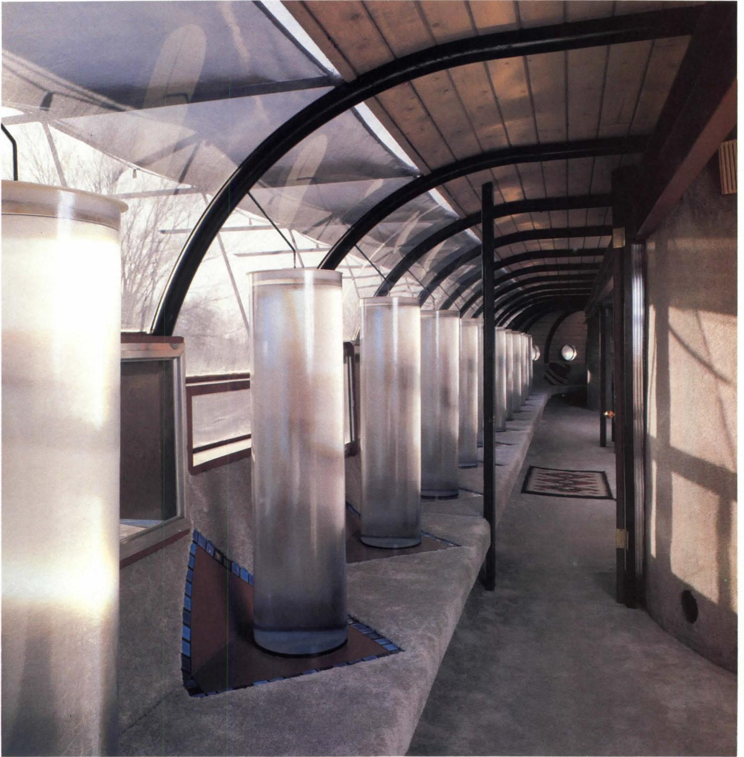
Structural steel I-beams support third-level bedroom quarters (below), which are clad in tongue-and-groove decking over custom-bent, three-inch-diameter metal ribs. By covering all walls and floors in monochromatic gray carpeting, Prince created a serene contrast to the more aggressive exterior—an effect that is heightened by light filtering through the translucent acrylic panels of a semicircular
