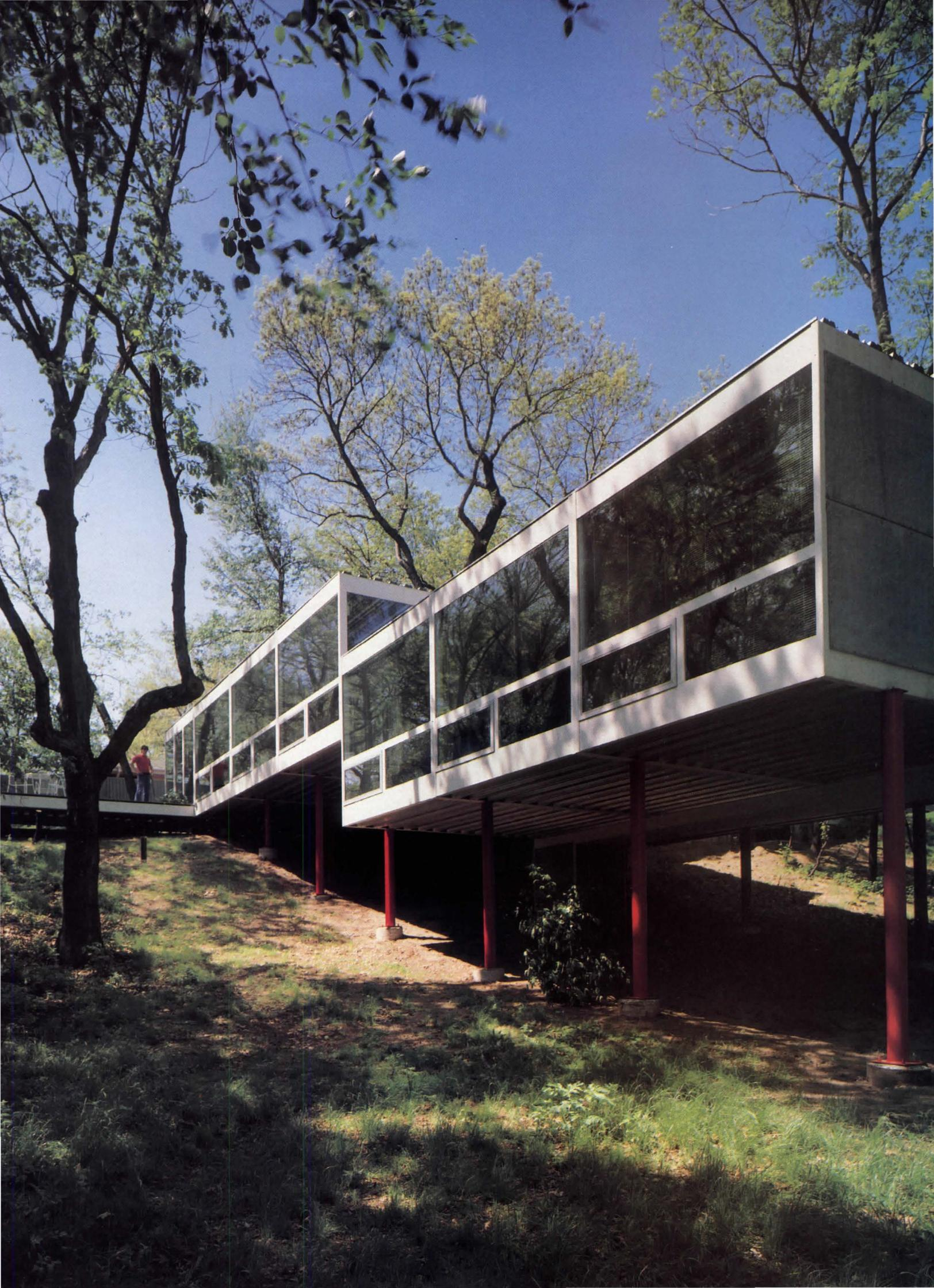
Stepping down with the hillside, the house lightly rests on lally columns set in minimal concrete foundations. The off-set of the levels also creates a bedroom "wing" and permits clerestory windows in the big open living-dining-kitchen area. A flat, modular steel unit forms a terrace for outdoor living off the dining area and convenient to the kitchen for serving. Utilities are banked into two "service cores," with
