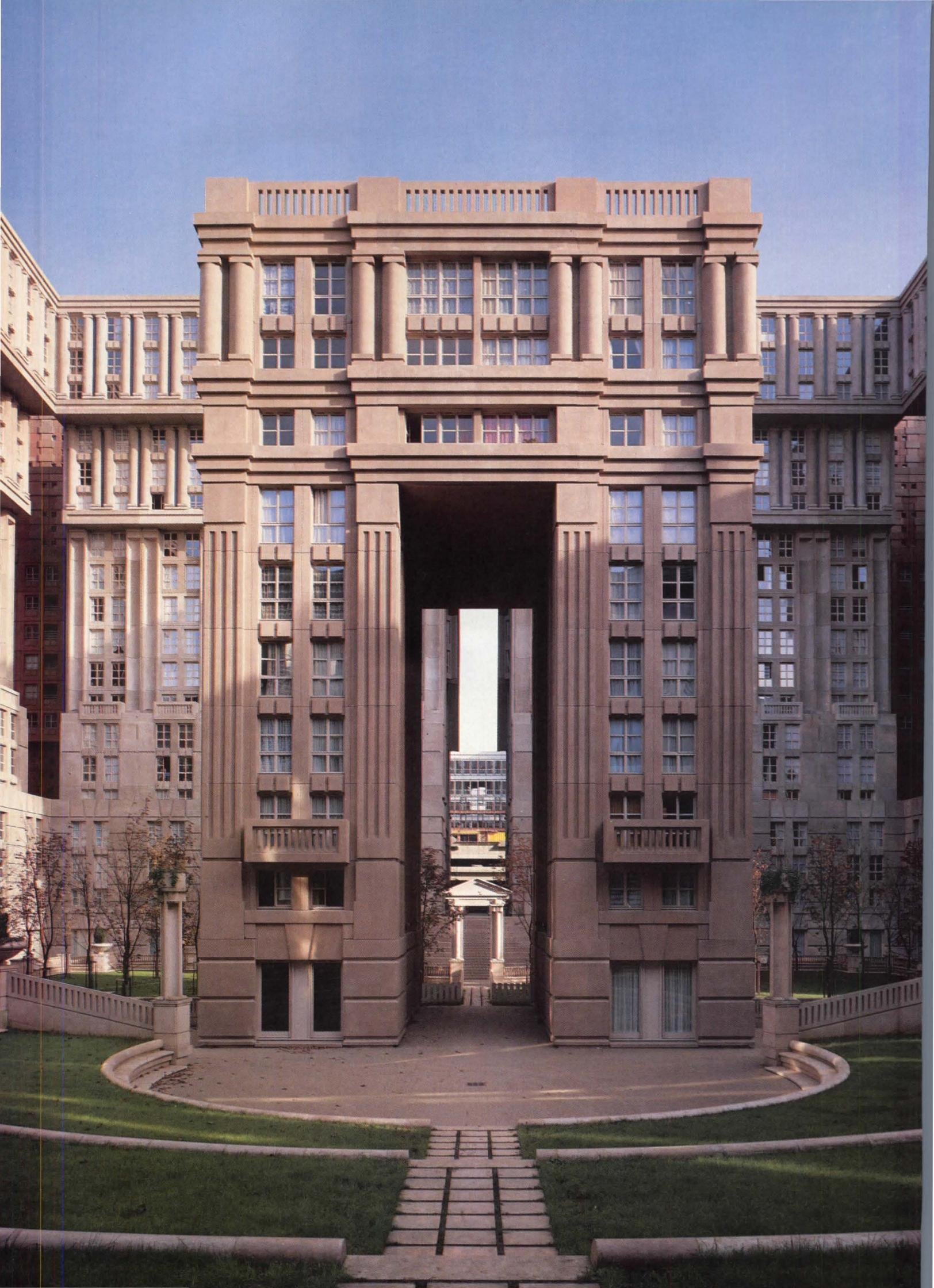
Many of the stylized, classical elements of Marne-la-Vallée are repeated on the triumphal arch and palace courtyard elevations, cast from the same steel molds (photo opposite page). All the stairs, arches, columns, balustrades and planters that furnish the courtyard are assembled from precast units and covered with an anti-graffiti, plastic emulsion paint. Sections through the cantilevered, exterior wall of the
