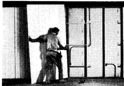
door, and glazing components that snap firmly in place for simple interchangeability.
