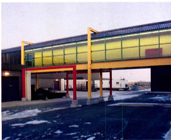
Vehicles are driven into Red River's auto shop through projecting vestibules to prevent the radiation of cold air into the interior (top photo). The building is connected to the rest of the campus by means of a pedestrian skywalk (photo above). South and north elevations are faced in glass (photo opposite), providing a view of the classroom mezzanine (left of section, opposite) and shop floor (right of section).
