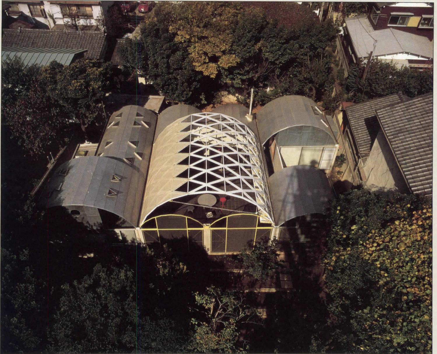
*The segmented axonometric at far left articulates the major elements of the construction system: concrete columns, steel beams, steel space frame, and flat-seam aluminum roofing with an interior finish of perforated asbestos-cement board. The end wall is infilled with perforated aluminum sheet metal. Lower drawing is a transverse section through the courtyard. The site plan, left, delineates the Silver*
