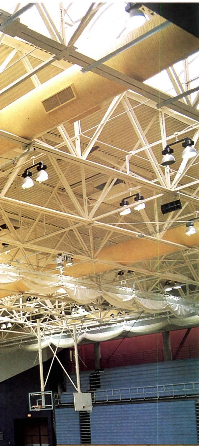
To build a sports complex as large and expansive as the Lund Center at Gustavus Adolphus College in St. Peter, Minnesota required a structural system that could go the distance. Vulcraft super long span joists were clearly the front runner.
