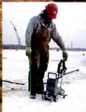
together with hot air for permanent seam integrity. Hot air welding is a simple, one-step process that can't be done with synthetic rubber roofs that require cleaning, priming, two applications of adhesive, adhesive set-up and finally bonding of the seams.
