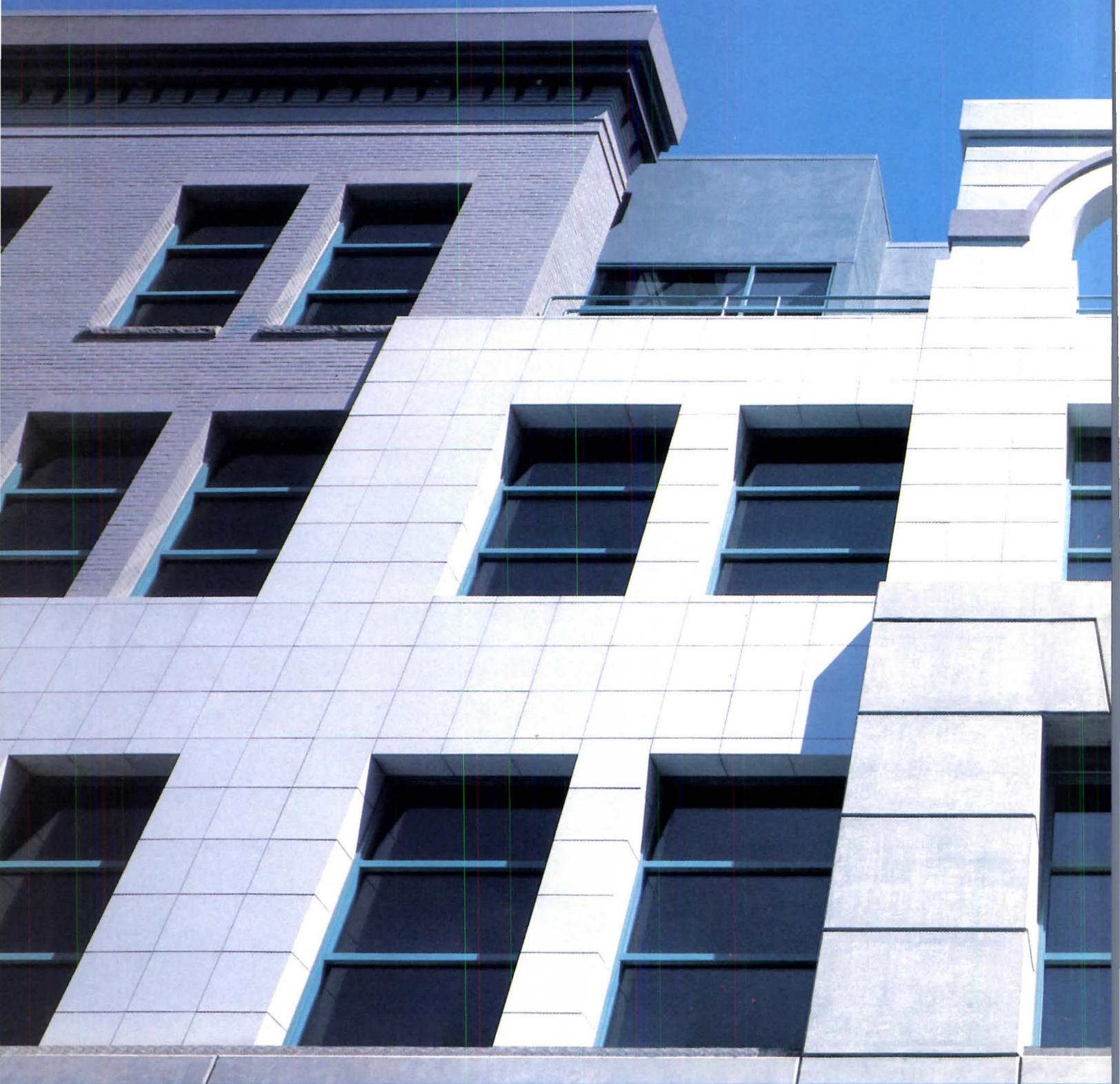
The remodeling called for a cladding material that would complement the terra cotta tile on neighboring buildings. It had to be easy to fabricate, easy to apply, and durable.
