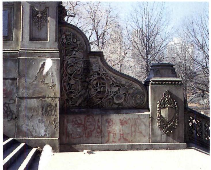
patch (left). A mixture of sand, lime, cement, water, and pigments in varying proportions was applied in three layers to achieve the proper depth (left diagram). Missing decoration such as birds' heads and trefoil cusps (top and bottom right) was replaced with newly carved sandstone replications to restore the original sculpted appearance. The new pieces were attached onto the old stone by
