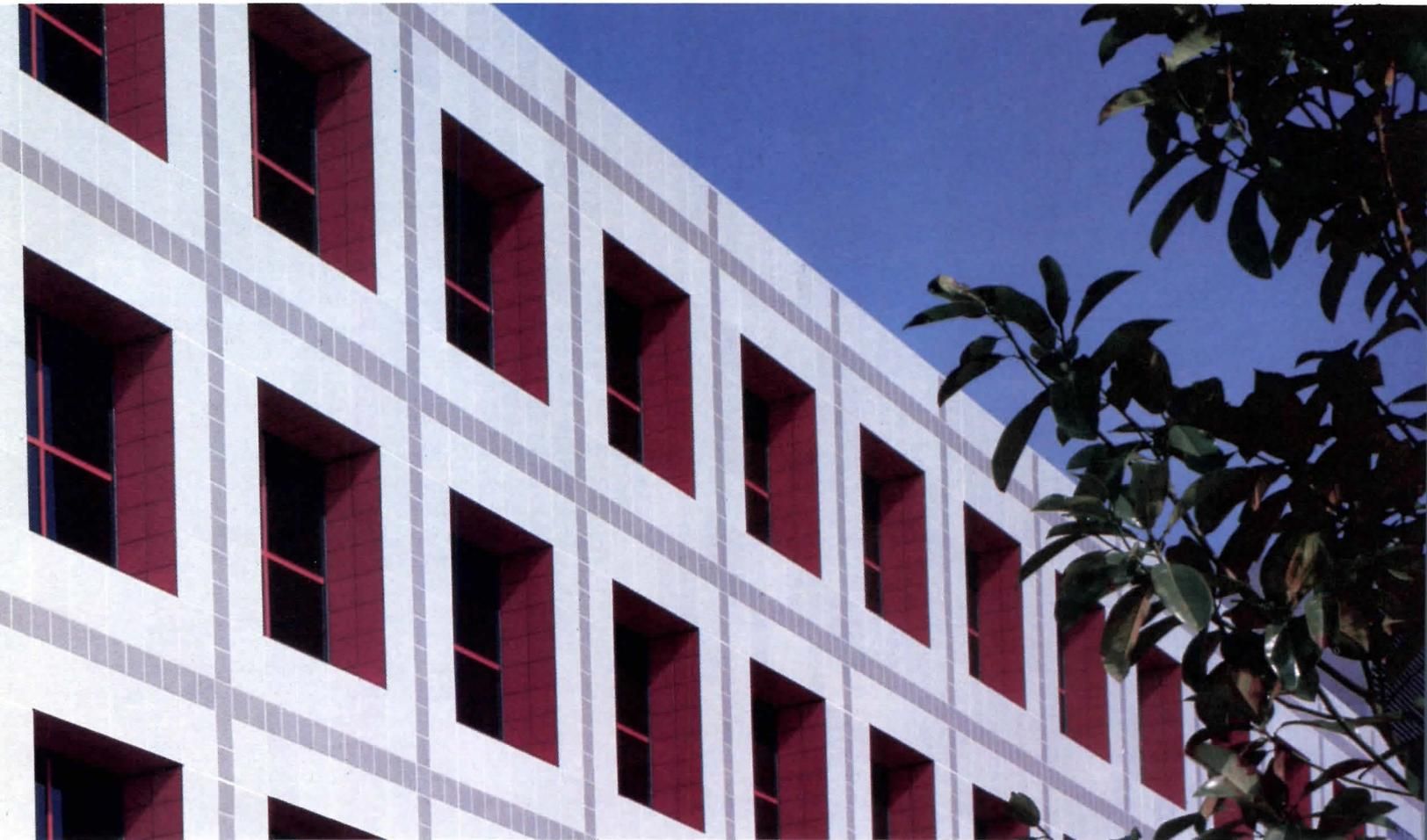
Exterior ceramic cladding. A design statement used by innovative architects to achieve enduring color, proportion, and resistance to weathering.
