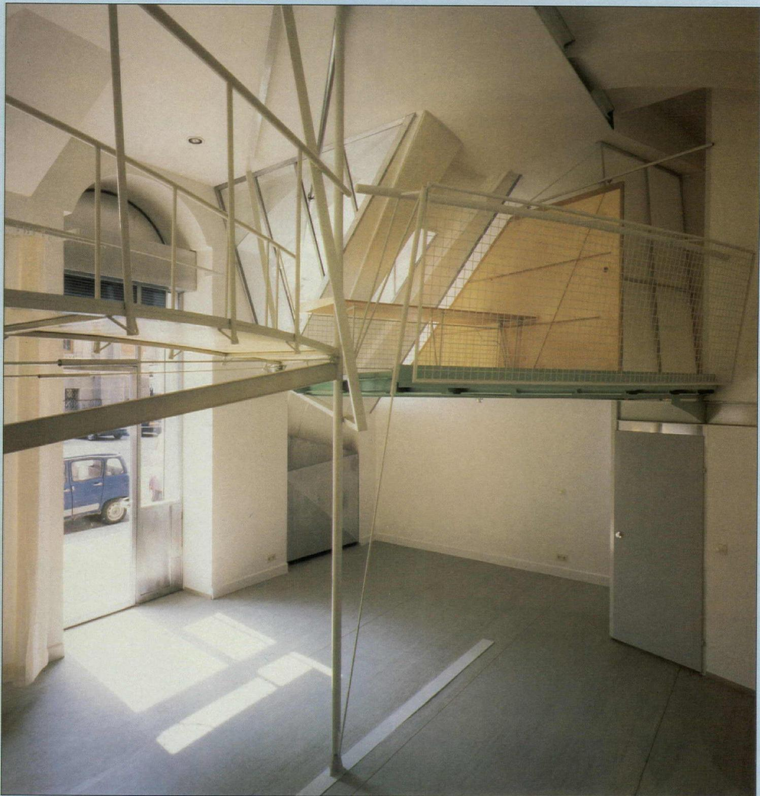
integrated into the walls to minimize intrusions into the ground floor working area. When the foldable steel stair is cranked to its "up" position (isometric drawing and photo this page), Baumann is left with a flying trapeze-like sculpture above his head. The architects painted the underside of the "office" a pale green (following pages), differentiating it from the rest of the white-coated steel
