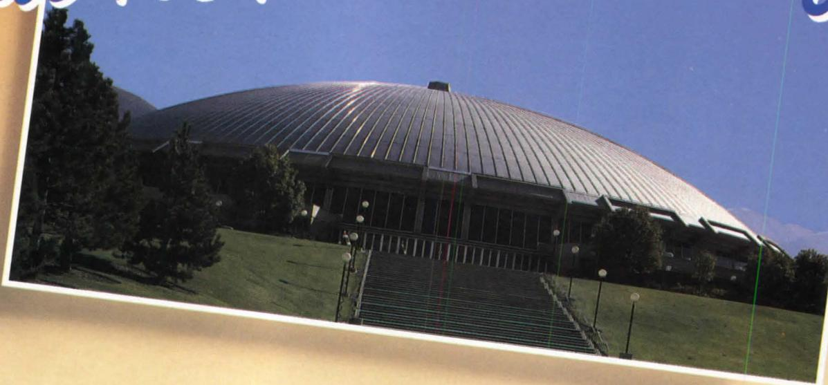
The original roof began leaking right after its installation on the Special Events Center at the University of Utah, Salt Lake City.
