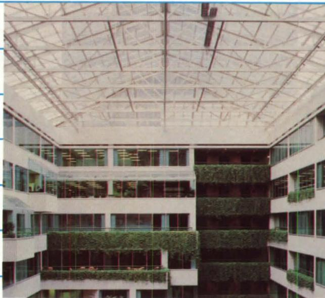
Architects list safety as a primary consideration in overhead glazing design. That is why laminated safety glass was specified in atrium of the Philadelphia Stock Exchange. In the event of breakage, laminated glass tends to remain
