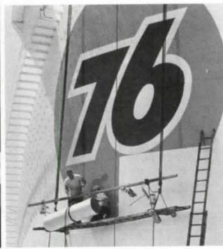
Flexible MODUCAL® decals with magnetic or adhesive backing can be used on flat or curved surfaces.
