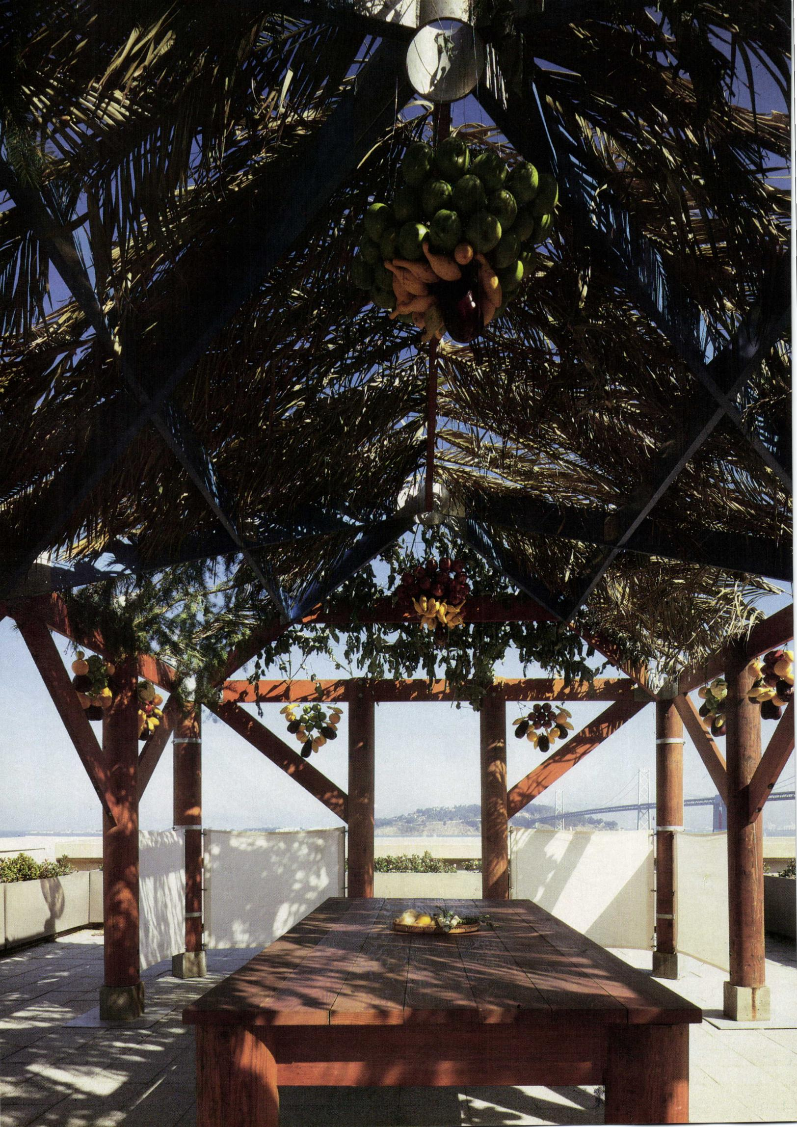
*Even though it is, by definition, impermanent, the sukkah must withstand wind and rain during its annual exposure on a San Francisco rooftop. Saitowitz incorporated four existing lampposts as structural anchors, to which 8-in.-diameter columns are bound with metal straps. Screws connect joist hangers and sheet-metal brackets for simple assembly and dismantling of the timber frame, which is hoisted onto the roof deck. Canvas panels lashed to the uprights lend shelter from the*
