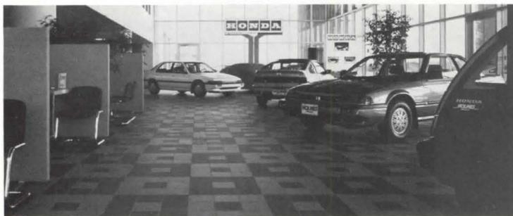
"The unglazed tile specified for the Holmes Oldsmobile/Honda showroom floor had to be extremely durable to accept the weight of automobiles," stated Bryan Shiffler, of Shiffler Frey Baldwin Clause Architects PC. "The owner was adamant about low maintenance, stain resistance and long life. It had to be impervious to showroom stains such as motor oil and gasoline and it had to be slip-resistant because of customers tracking in snow and ice. It also had
