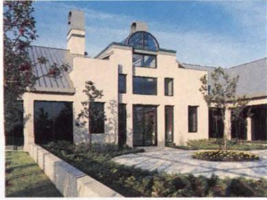
A major unifying element throughout this mixed use development, is the choice of Dryvit exterior insulation and finish system (EIFS) for exterior walls. Towering chimneys of Dryvit EIFS further unify the whole, while making a strong design statement of their own.
