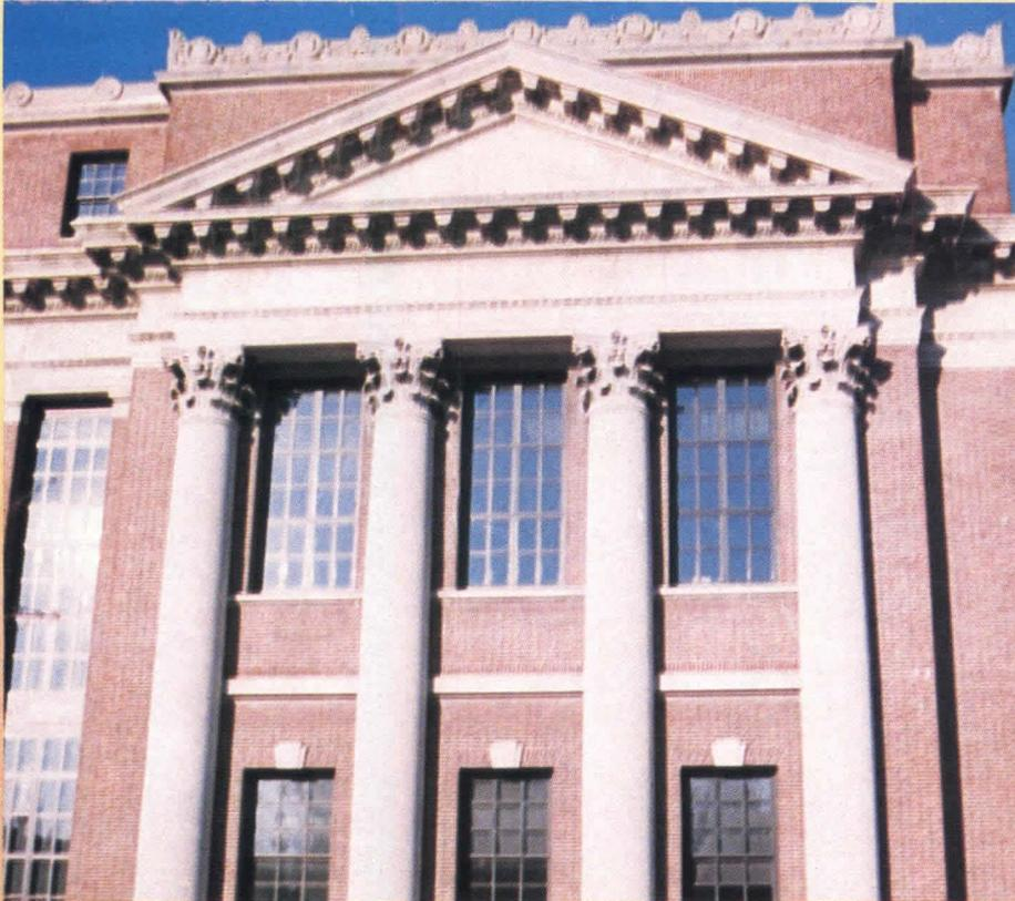
**Widener Library, Harvard University.** Original casement, awning and fixed windows were reproduced. Precise physical dimensions and projections for all profiles were maintained within 1/32 of an inch as specified.
