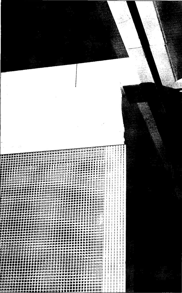
*Though formed of seemingly simple, familiar hardware that might have come from the shelves of the local building-supply house—steel-framed perforated-metal panels suspended from an overhead channel/grid—SITE's floating wall system achieves refinement through painstaking engineering and craftsmanship, abetted by classical cornice and base moldings that recall the historic roots of its setting.*
