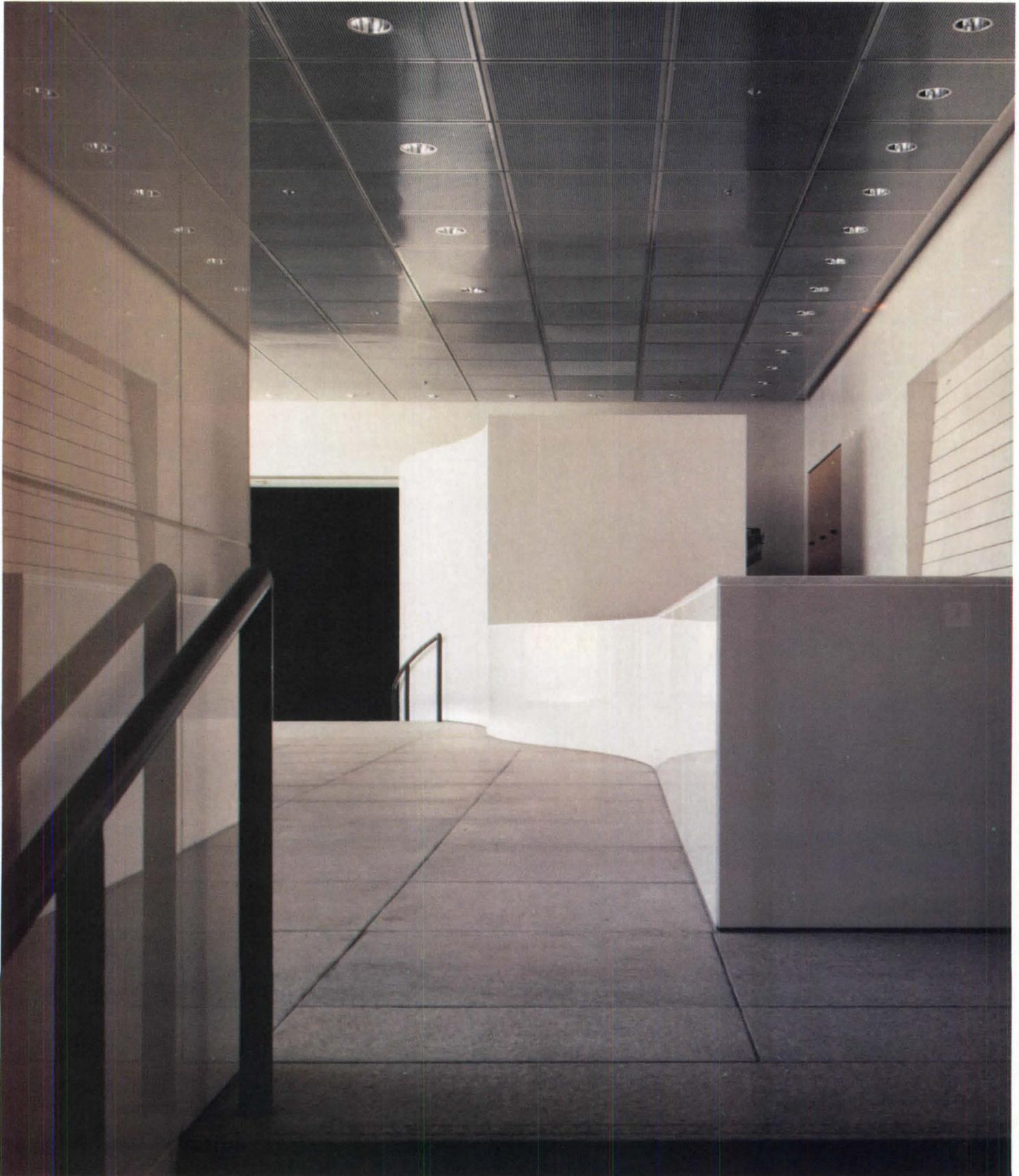
perforations serve for both air supply and return. The trim, reflectors for recessed downlights, and the sprinkler heads were selected to coordinate with the aluminum of the panel—a milled material with a clear lacquer coating. Perforated metal
