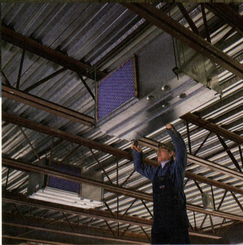
*5-foot spacing between Vulcraft joists permits easy installation and maintenance of heat pump units.*
