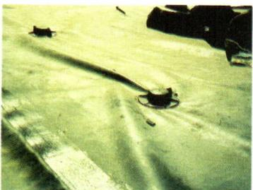
*distributes stresses caused by wind uplift. The non-penetrating attachment in fig. 6 shows the membrane movement caused by the wind, which can result in seam failure (fig. 4). Wind uplift can also redistribute ballast (fig. 5), leading to roof failure.*
