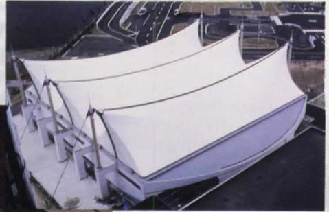
Point-hung tensioned membrane structure at Toyohashi.
