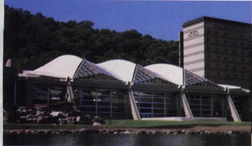
Glass gables are integrated into Sun Palace membrane roof.
