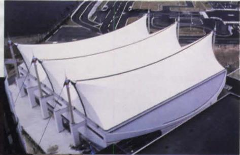
Point-hung tensioned membrane structure at Toyohashi.
