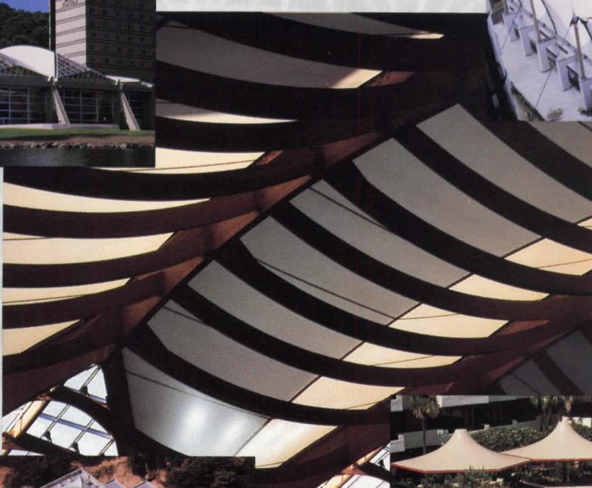
Glass-laminated wood structure supports tensioned membrane roof at Sun Palace swimming facility.
