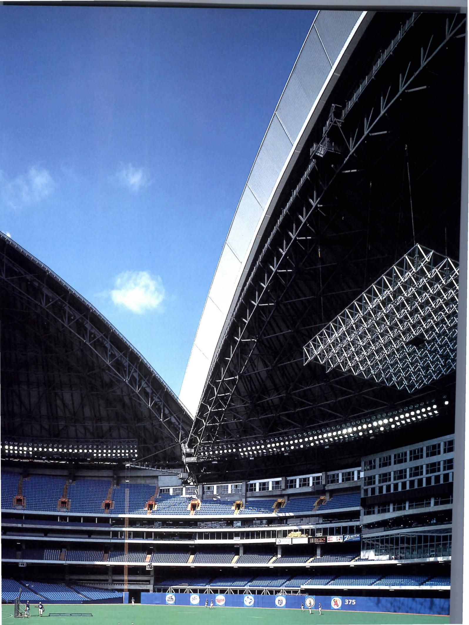
In the roof's closing sequence, Panel 1 rotates 180 degrees from behind a fixed shell (1, 2) to a position at the southern end of the stadium (3). Once it is clear, the transverse-vaulted Panels 2 and 3 begin moving on parallel tracks to seal the gap (4).
