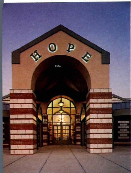
Restricted to a \$4.5-million construction budget (\$83/sq ft), Taft Architects used a 60-foot-wide repetitive steel frame and inexpensive materials such as brick and concrete block. The architects tied the new elementary school to an existing high school and playing fields by superimposing a grid of pathways and trees on the property (site plan below). A major design feature is the school's indoor "main street," which is lined with brick-and-concrete arches and pyramid-topped pavilions.
