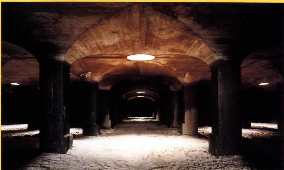
re concrete compartments (bottom right) partially filled with sand. Filtered clean water was funneled to an underground reservoir, where it would remain until the pumping station distributed it throughout the city. Soon after Hazen's silos and regular houses were put to use, Frederick Law Olmsted, Jr., was hired to make the surrounding area more inviting to the public. Instead planted allées of mulberry trees along pathways between the silos and regular houses, transforming the blanket of
