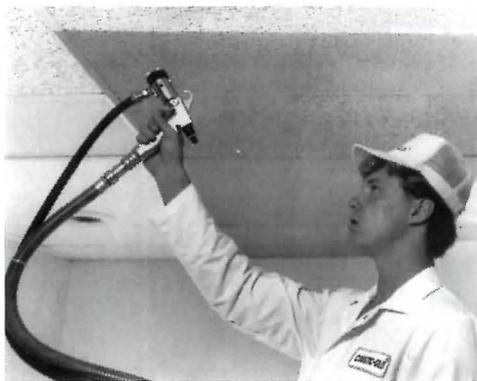
**312. Ceiling-tile coating.** Cooustic-Coat is a cosmetic resurfacing material that is sprayed on acoustical surfaces. Available in six white and off-white shades, the water-based vehicle can also be tinted to match any color. Said to leave the pores and fissures open, it will not bond panels to grid. The coating meets California State Fire Marshall flame-retardant standards, and will not compromise the flame- and smoke-ratings of a rated ceiling. Cooustic-Glo International.
