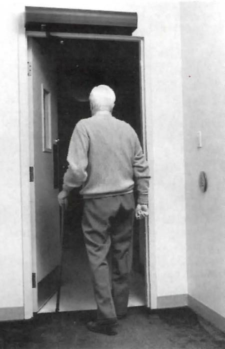
**16. Door operator.** Gemini GT operators provide the option of both manual and automatic access. They are suggested as an economical retrofit (under \$1,000) to make doors accessible to the elderly and handiapped. All components are surface mounted for easy installation on existing doors. Both hold-open delay and opening speed are adjustable. Gyro Tech, Inc.
