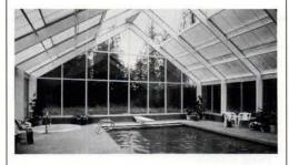
**342. Pool pavilion.** The Classic 2000 glazed enclosure has a roof of insulating Danpalon translucent panels dry-glazed within a motorized retractable-roof system; in this application, the panels move downward from the ridge. Perimeter walls are glass. Clear Plastics International, Inc., Mundelein, Ill.
