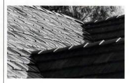
**317. Replica roofing.** A new roof tile is made of an A-label composite plastic, formed in molds taken directly from natural slate and cedar shakes that produce a distinct, realistic texture. Molds and colorations vary from tile to tile, giving a random effect to the installed roof. Individual tiles interlock for added wind resistance, and take foot traffic without damage. Everest Roofing Products, Walnut, Calif.
