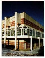
Reynobond®FR Aluminum Composite Panels were utilized as spandrel panels, fascia, soffit, column covers & truss beam wrap on the M.I.T. Lincoln Laboratory Facility. Reynobond®FR is the only solid thermoplastic core composite panel whose core material is categorically inert, non-toxic & fire resistant. Case history available with supporting data. Reynolds Metals Co., P.O. Box 27003, Richmond, VA 23261, 804-281-3629.
