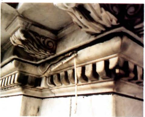
3. Water penetration at the foot of the stone portico column has corroded the brick-arch support beam, and the rust, having much greater volume than steel, has pushed up against the column base, breaking its corner.
