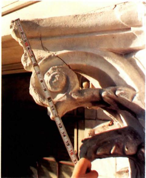
2. This crack was filled with sealant. The stone should have been repaired by injection of a bonding agent (sealants' adhesive bond with stone usually fails shortly after installation). Better yet, it should have been replaced.
