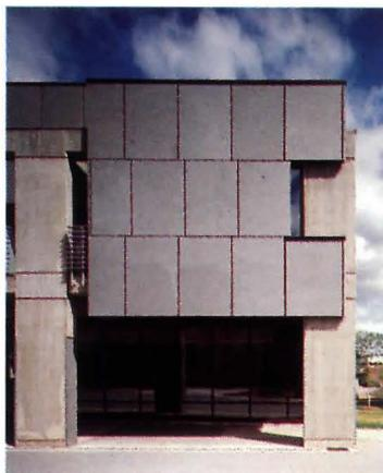
*To economically add lounges, offices, and food-service areas to an existing student center, Kieran, Timberlake & Harris wrapped the brick-clad original with a small addition to the south and a larger addition to the north (drawings above). The wall expresses its layering of cast-in-place concrete frame (which forms an arcade on the north side, opposite and left), suspended open-joint granite panels, and windows set in the backup wall (above).*
