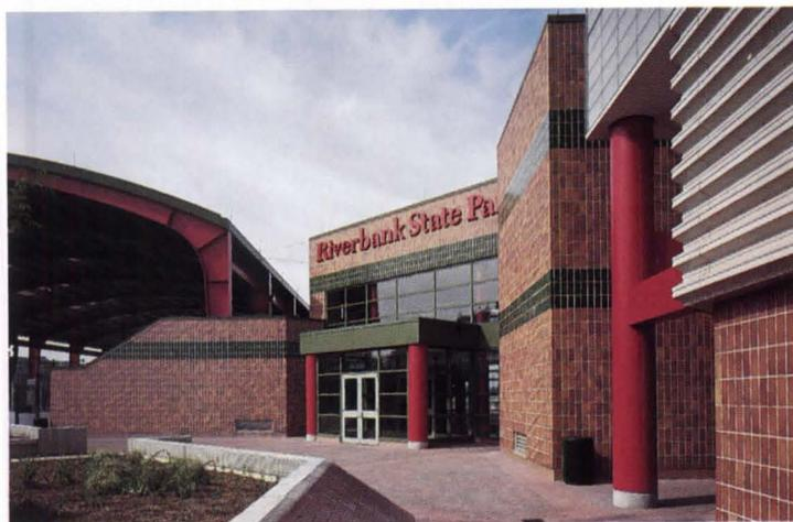
*Three views of the Cultural Building (top left and right), and the main entrance to the park. Because all building loads had to be transferred to columns that rested on columns supporting the plant, Dattner chose lightweight tile-and metal-faced panels as the primary wall system. The roof structure of the skating rink is visible to the left of the Cultural Building entrance.*
