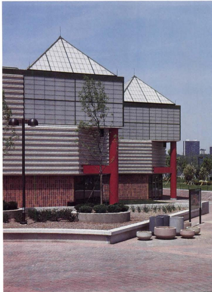
Three views of the Cultural Building (top left and right), and the main entrance to the park. Because all building loads had to be transferred to columns that rested on columns supporting the plant, Dattner chose lightweight tile-and metal-faced panels as the primary wall system. The roof structure of the skating rink is visible to the left of the Cultural Building entrance.
