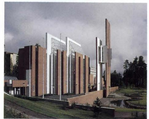
*The 114-foot-high bell tower is composed of two vertically cantilevered concrete slabs. Just above mid-height, a series of horizontal and vertical planes form a box to stabilize the two primary planes. Slender white ribs projecting from the red brick stiffen the upper part of the main tower panel.*
