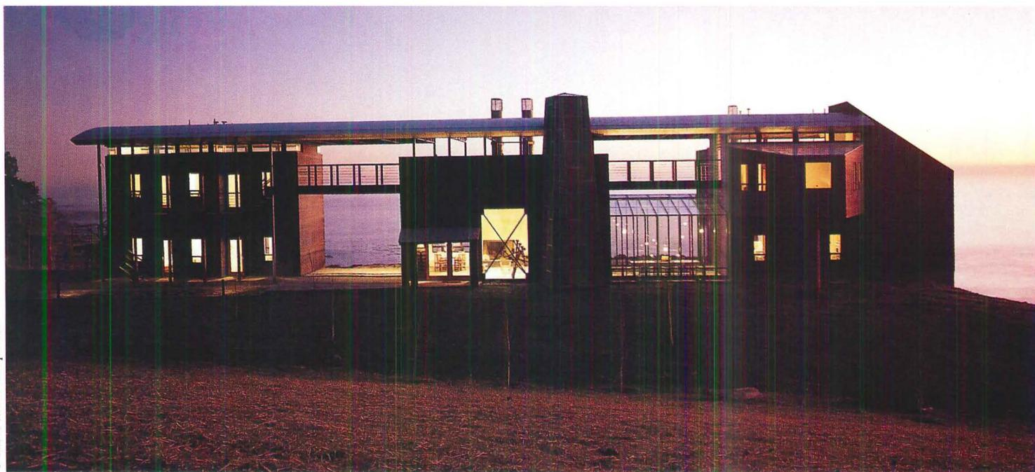
*Heavy winds, the weight of up to 300 guests, and brush fires were among the design problems. An extra-heavy structure and a galvanized-steel roof over rigid insulation were the solutions.*
