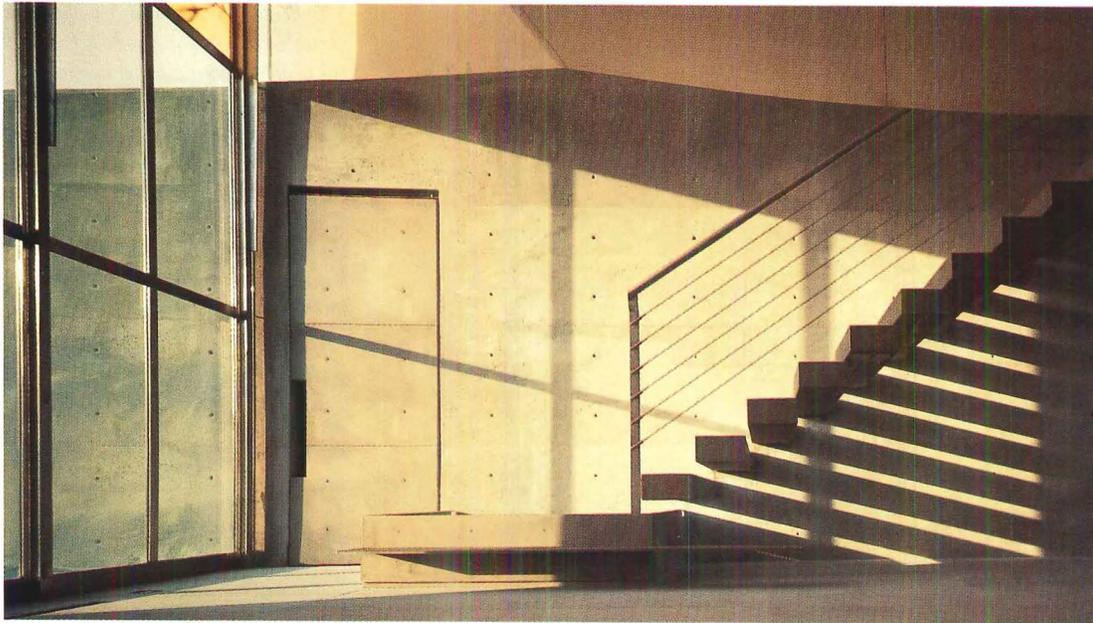
Zapata and West used stainless steel in three forms (wire, beaded and polished) throughout the house. Concrete stair treads were covered with beaded stainless; the railing is polished steel strung with wire cable. The door to the kitchen is also beaded stainless steel. In many cases, poured-in-place concrete walls were left untouched. In the foyer, the floor is the same blue-green serpentine used on the terrace and pool coping. Other floors are covered in mahogany, maple, and sisal.
