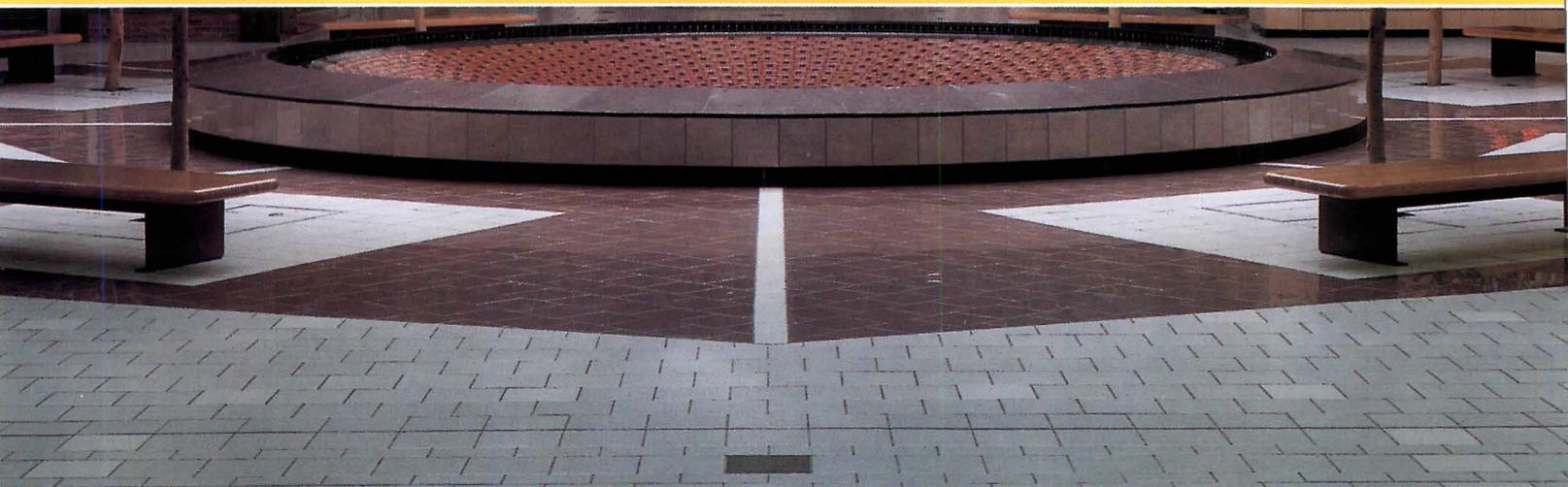
Five new porcelain pavers with water absorption rates of almost 0%. And breaking strengths that double the ANSI standards.
