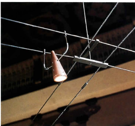
Located in a landmark building where no new ceiling- or wall-mounted fixtures were permitted, the exhibit has been lit with the aid of cables connected to poles standing on a built-up floor. The cone-shaped fixtures use MR16 lamps with UV filters to protect the fragile artifacts.
