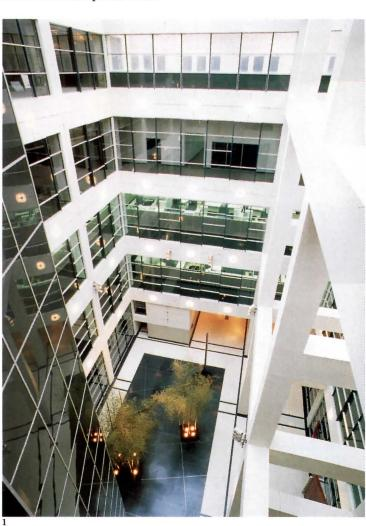
The original heavy-duty column-and-beam construction is expressed in the atria (1), where it stands free of enclosing walls. Under the glazed roof, old steel hoist beams painted with zinc-chromate primer recall freight elevators that once filled the space. Existing 19-foot ceilings on upper floors (2) are ideal for large drafting rooms. On the main floor; 22-foot ceilings allow extra offices on mezzanines (3).
