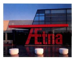
includes a redesign of the site to soften the typical mall's bare parking lots with perimeter trees and landscaping around the building; a 2,400-square-foot curving addition to modulate the original store's high-bay bulk; new tinted-glass curtain walls around the entire building perimeter and a new glass-roofed courtyard to bring outside light into once windowless spaces; and an upgrade of all building amenities, such as
