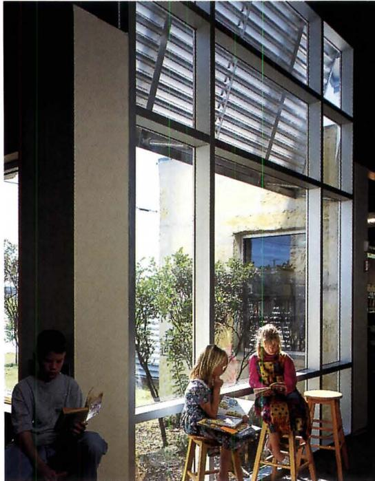
Although the library is just one big room, there are comfortable, quiet places to sit and read. The glazed end walls of the high bays are recessed back from the stone enclosing walls of the low bays, forming mini-courts around which seating is placed. The high bays are also pleasant to sit under since the book stacks and perforated roof decking system soften the acoustics.
