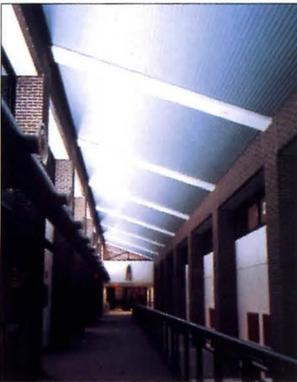
LUXALON<sup>®</sup> Linear Metal Ceilings, a Hunter Douglas product, are prominently displayed at Harper College in Palatine, Illinois. A Wide selection of profiles and carrier options offer complete design flexibility. 130 colors, ROUND EDGE, SQUARE EDGE, and V-GROOVE (featured) profiles enhance both the design and acoustical performance of any space.
