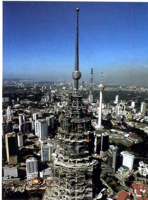
*At the Petronas towers (above), high-grade concrete and self-climbing forms helped erect the world's tallest buildings faster.*
