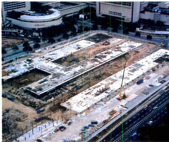
*In the top-down construction used at the Singapore International Convention and Exhibition Center (left and drawing above), the ground-floor slab was built in an E shape, which allowed excavation to the first basement level to be done mostly in the open*
