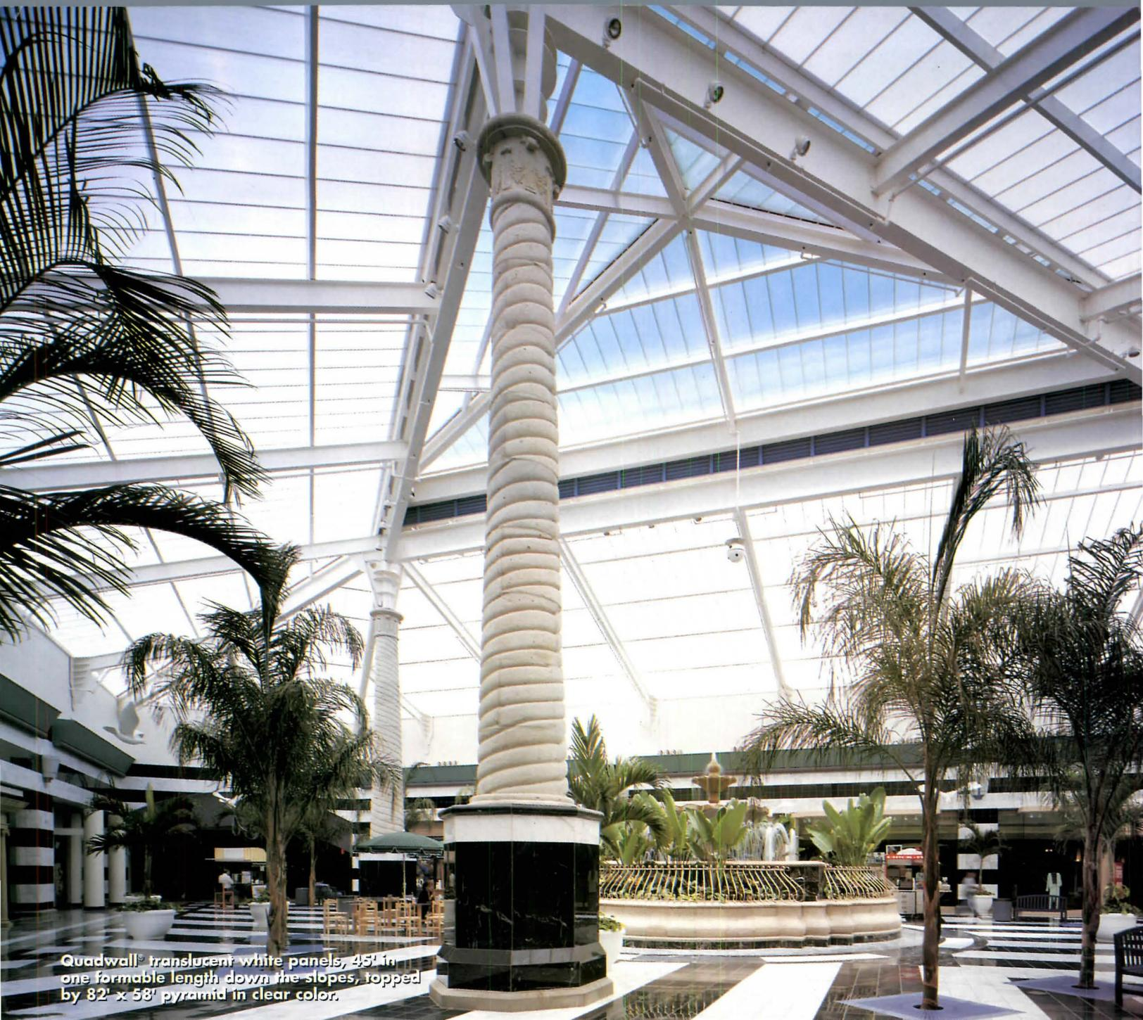
Quadwall® translucent white panels, 45' in one formable length down the slopes, topped by 82' x 58' pyramid in clear color.
