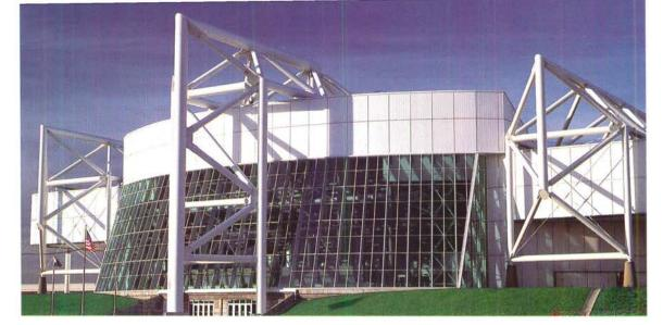
Product: EFCO Series 5800 Silicone Gasket Curtain Wall System (formerly Don Reynolds Curtain Wall System)
