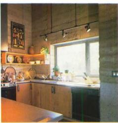
Views of a rammedearth house (left) show the horizontal banding that occurs when layers of soil are placed in forms and pneumatically compacted. Only some types of soil are suitable for the process; also, rammed earth will not hold up in damp environments.
