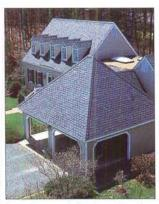
has been sheltering America for over two centuries. As a roofing material, it is prized for its high mica content, natural cleft and texture, as well as its non-fading and distinctive handmade quality. Because of it's permanence and natural beauty, it was specified by Thomas Jefferson in the 1800's and remains today the roofing choice of eminent architects. Buckingham-Virginia Slate, P.O. Box 8, Arvonia, VA 23004. T: 1-800-235-8921.
