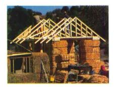
Straw-bale walls are topped by a timber roof structure (left) before being finished. Because the walls are typically 18 to 24 inches thick, deeply set windows (below) are necessary.
