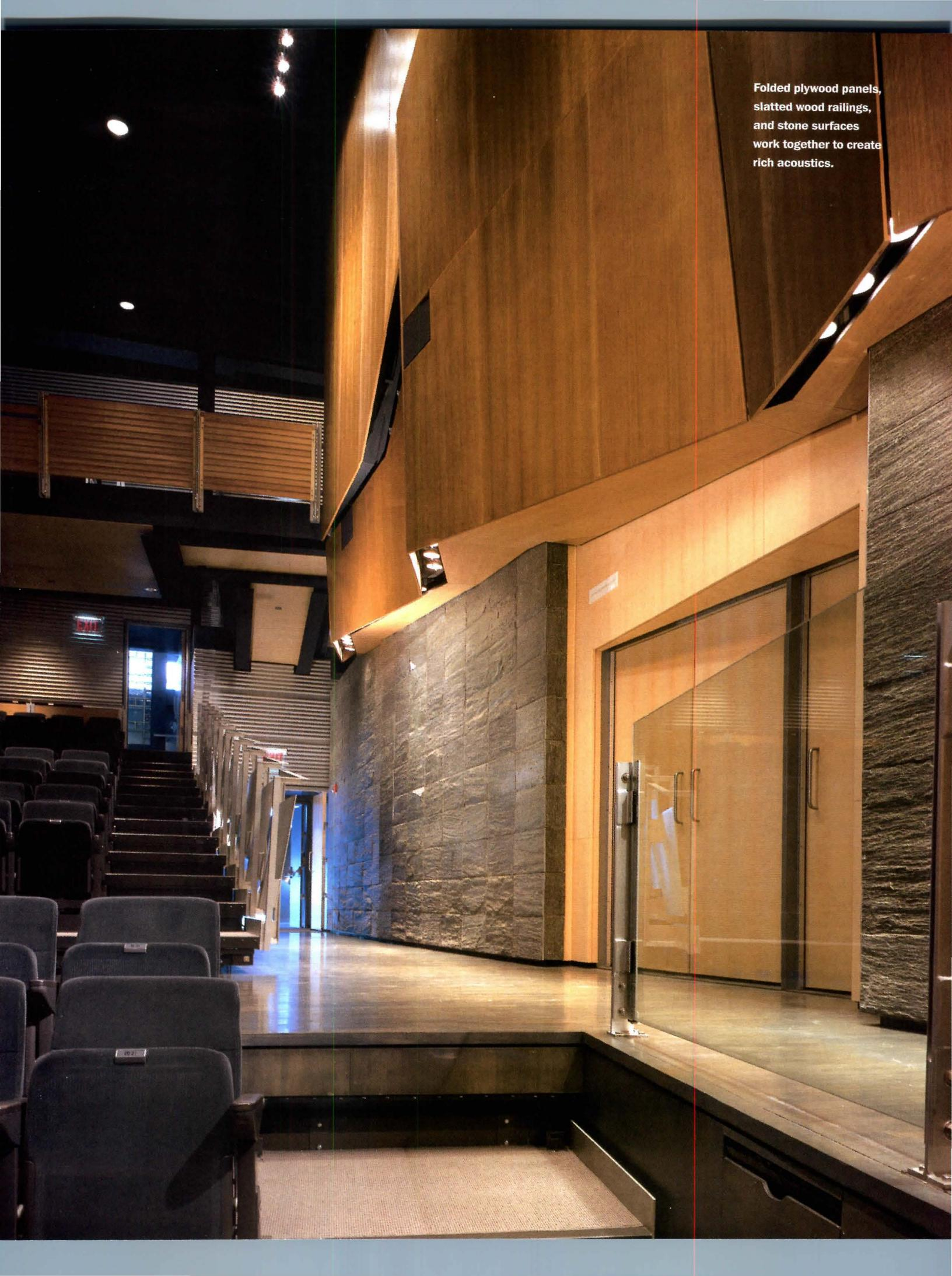
Folded plywood panels, slatted wood railings, and stone surfaces work together to create rich acoustics.
