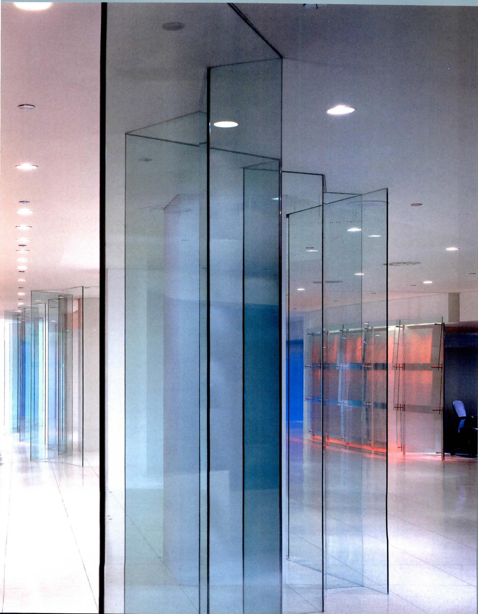
The front zone of the showroom (opposite and right) was intended to convey Herman Miller's credo of openness and flexibility. Circles sandblasted on both sides of the partitions' glass panels are meant to provide some privacy without completely sacrificing translucency.
