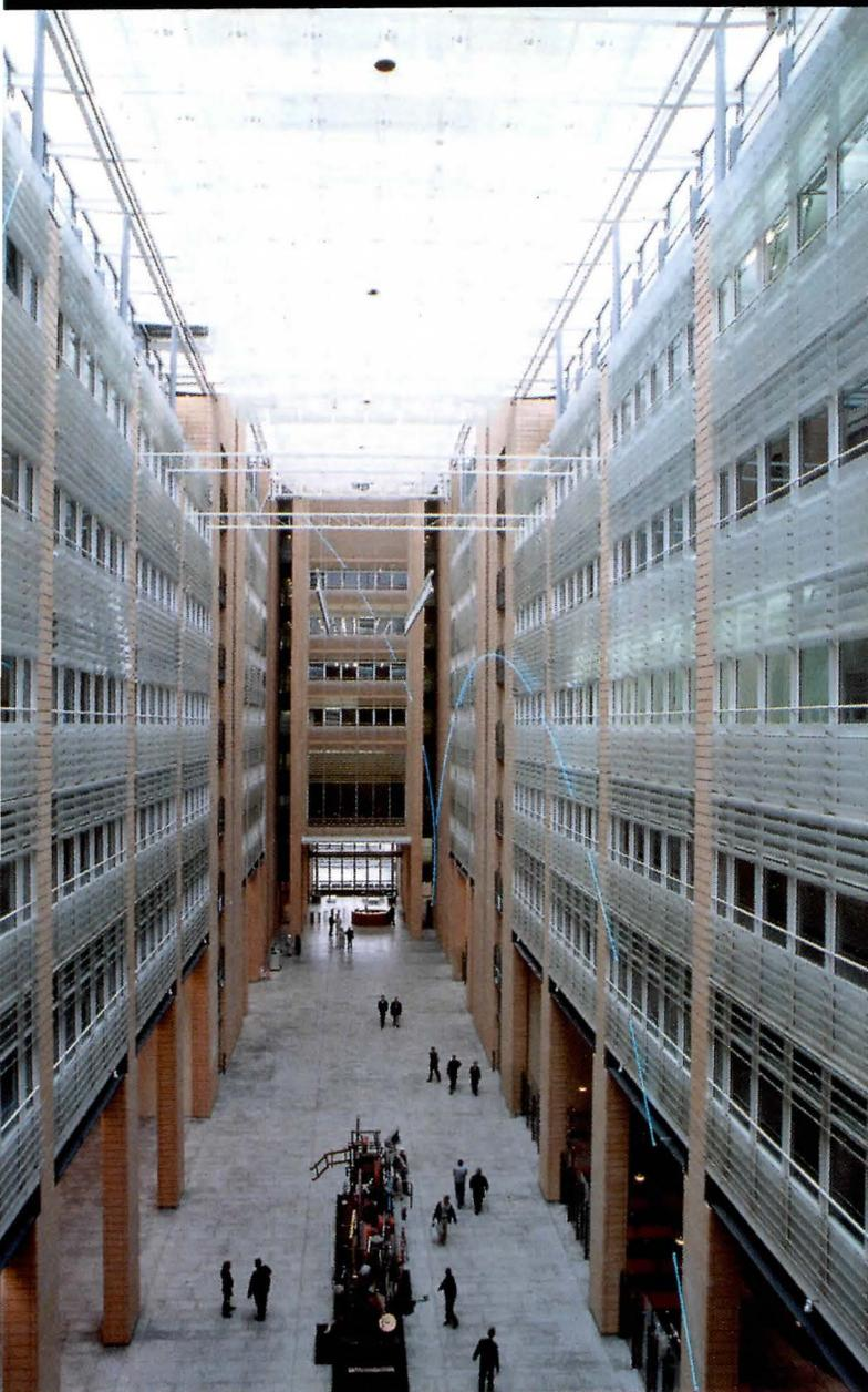
Though the atrium is vast (looking south this page, north opposite page), the diaphanous quality of the skylight system and the solar-protection fins (right) visually dissolves the space's borders.
