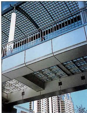
offers structurally engineered, prefabricated monolithic Glass Panel Systems. Preglaced & fully waterproof frameworks of Aluminum, Precast Concrete, Steel & Cast Iron incorporate Hollow Glass Block, Solid Glass Pavers, Glass Bullets & Plank or Insulated Glass. Standard & custom panel sizes are available for installation as windows, walls, flooring, stair treads & landings, bridges, sidewalks, skylights, complete structures or virtually any application. 1-800-358-3888
