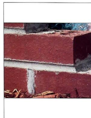
are inexpensive and easily installed in weep holes to insure masonry cavity walls breath, drain and dry quickly. Made from 100% recycled polyester with a 90% open mesh in 2.5" x 4" x .5, they are available in white, tan, almond, gray, and brown. Weep Vents add to the beauty of the wall by duplicating the texture and color of mortar, thus eliminating open holes and dark shadows while restricting entry to insects. Call (800) 664-6638 for more information.
