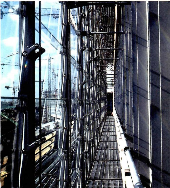
At the southern end of the building, Piano peels away the successive layers of the curtain wall, revealing outer pivoting glazing, the outer-wall support
