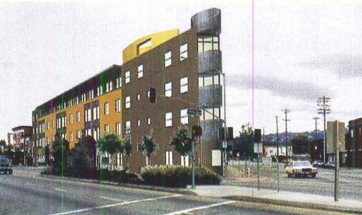
been inappropriate for a civic-scaled street,” explains Massih. The design reduces the scale and “keeps it from looking too institutional and old-folksy.” A single 90-foot bay of wood siding, painted yellow, encases three four-window blocks set into corrugated steel.
