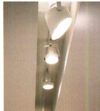
Monopoints can be plugged in along the beams wherever they are needed (top). A channel in a ductwork soffit hides track lights (above).
