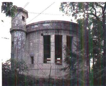
A construction view of the cistern's north elevation (left) shows the existing stair tower and new double-height window openings. Bay windows with aluminum mullions painted black were added on the east face (below). On the south side, a trellis is visible from below (opposite, top left and bottom).
