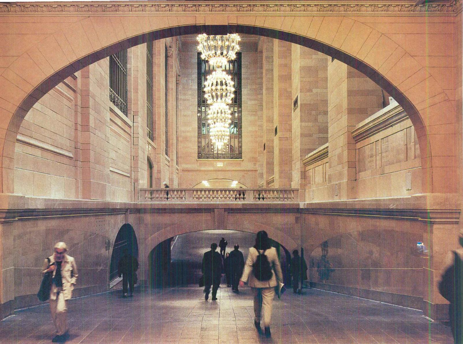
Removing offices added in 1927 over the ramps leading from the Main Concourse to the Lower Concourse has turned a tunnel-like corridor (left) back into a dramatic space (right). The architects changed the bridge over the ramps (above), designing a new balustrade that offers views down. The bridge originally had an eight-foot-high wall that shielded long-distance travelers from seeing commuters below.
