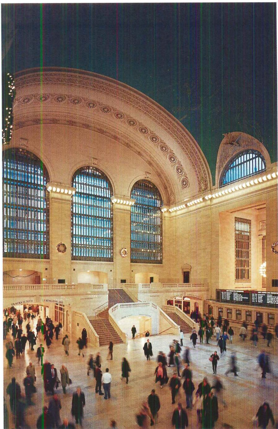
The terminal's arched windows (left and below) each measure 33 by 60 feet and form a double skin of glass. Glass walkways run between the two transparent skins, connecting offices on either side. A new east stair (left) stands where the Kodak sign used to be and provides access up
