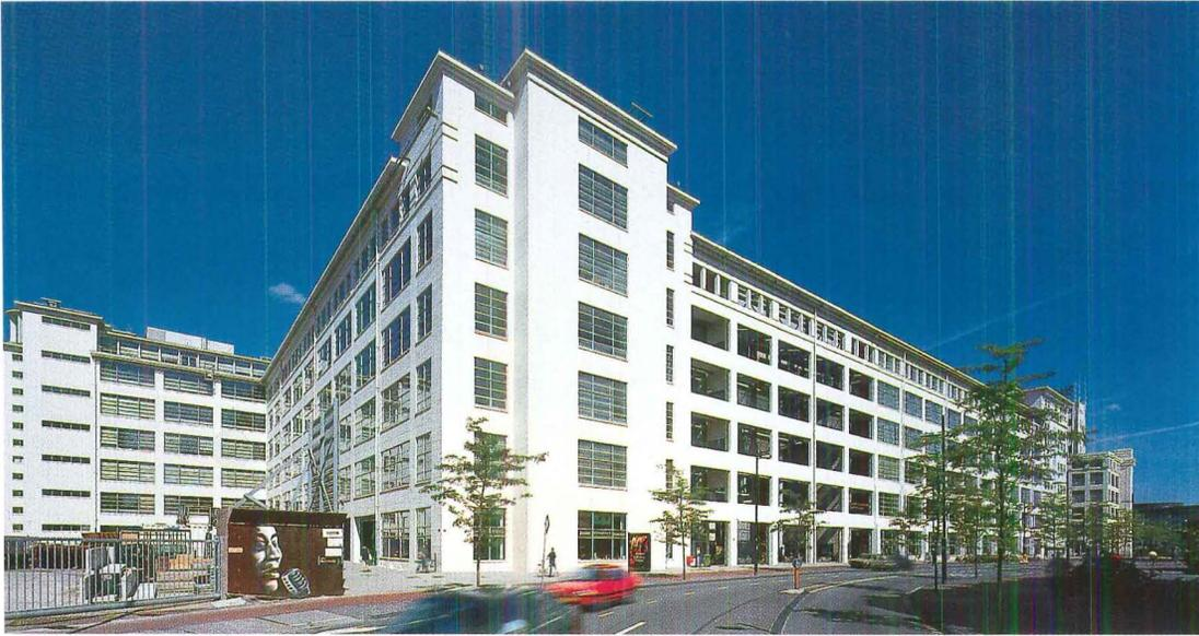
The building's fenestration was changed from small-paned windows to large double-paned expanses of glass (left). The Light Plaza (below) offers Philips a place to show off some of its outdoor lighting applications.
