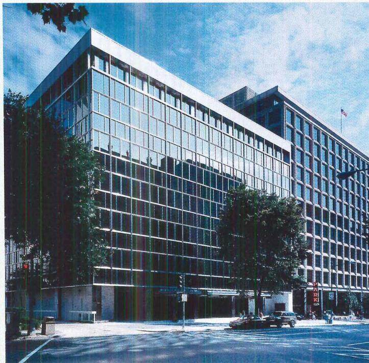
window system was permanently closed and inch-thick insulating glass was used to replace the original ¼-inch glazing. The original metal spandrel panels were replaced with glass to match the glazing elsewhere. In so doing, at least one design compromise was made: the original horizontal banding was eliminated. “But it could be put back
