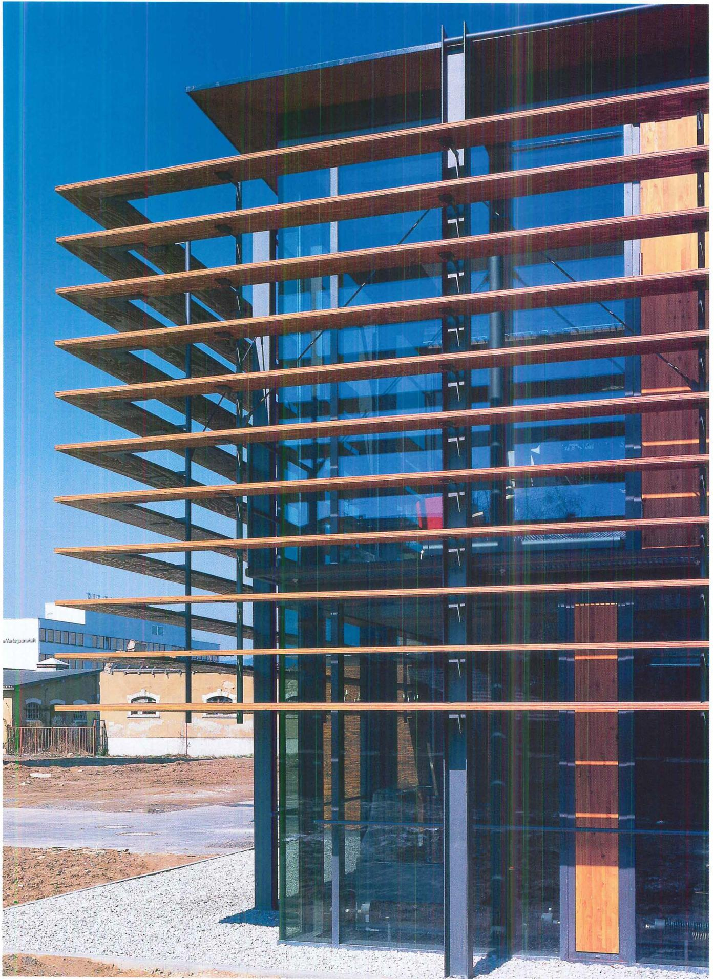
A steel structure supports the curtain wall, as well as Nordic-pine plywood louvers, which allow for transparency while shading the interior (right, below, and opposite). Louvers are set two feet from the face of the glass to provide minimum width for a second-story fire escape. Lamott gave the louvers opened-ends fins (below and right), instead of wrapping the entire building. Befitting a library, the interior is legible from outside.
