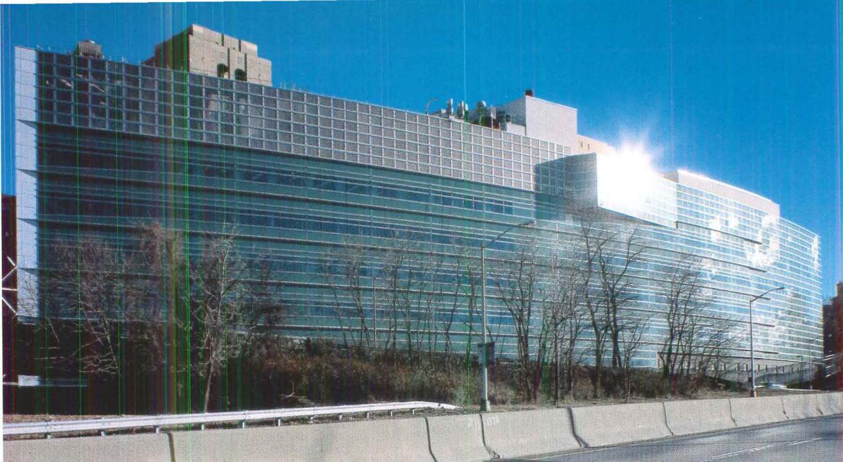
materials: Precast concrete panels for inpatient rooms, glass curtainwall for activity areas, and aluminum panels for support spaces.
