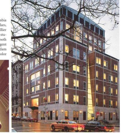
A prismatic light guide makes a Warren Hall's glass-enclosed stairwell a nighttime beacon of light.
