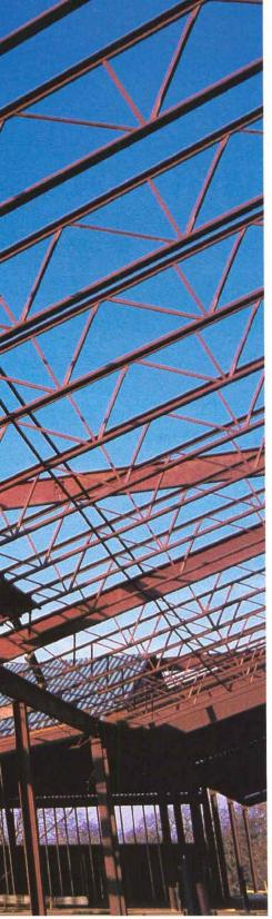
Take a lesson from the Bransford Elementary School in Grapevine, Texas. Where the structural engineer saved money using Vulcraft sloped seat steel joists instead of wood construction
