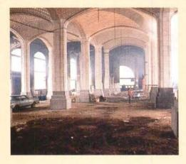
dimension reputedly determined by the largest size a mason could pick up in one hand. Applied in a basketweave pattern, the tiles were capable of spanning greater distances at a lower rise than stone. Furthermore, the company's total control over the design, production, sales, and installation of its tiles increased the speed and economic viability of construction.
