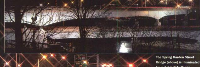
The Spring Garden Street Bridge (above) is illuminate by metal-halide floods mounted on the banks of the river and along West River Drive.
