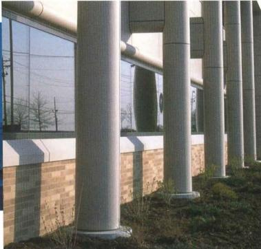
Thermoforming, the process in which plastics are heated and shaped, created additional design possibilities, says Warner: tight-radius curves for column caps, intricate bullnoses, seamless beam covers.
