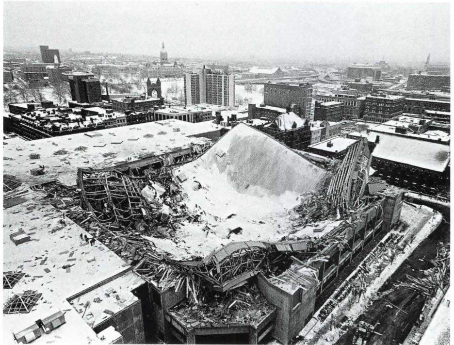
The roof of the Hartford Arena collapsed in January 1978 under the weight of a heavy snowfall.
