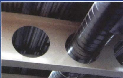
Electrical and mechanical services run through rather than under reducing floor to floor heights; therefore reducing costs of your structure.
