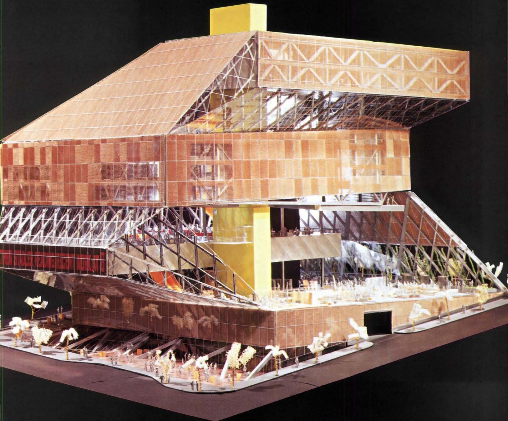
Blocks of floors shift toward views and light inside a diamond-patterned mesh woven by I-beams and steel tubes cloaked in a glass curtain wall. Alternating
