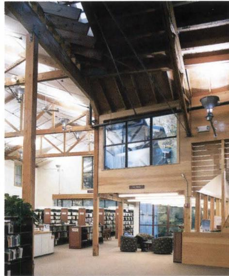
The lobby's splayed walls push its ridge line uphill to intersect with the reading room's gable roof (this page and opposite). A skylight filters sunlight through multiple layers of framing members.
