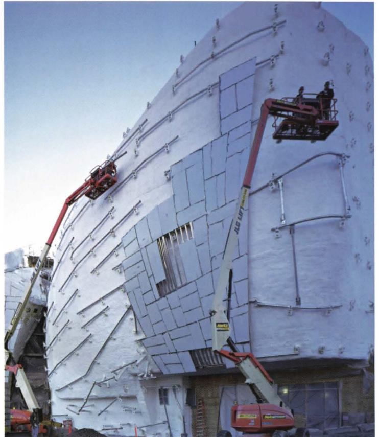
Five-inch aluminum pipe girts, which could be adjusted four inches in any direction at either end as required to locate them precisely, were first anchored to structural pedestals. Next, the metal panels were installed.
