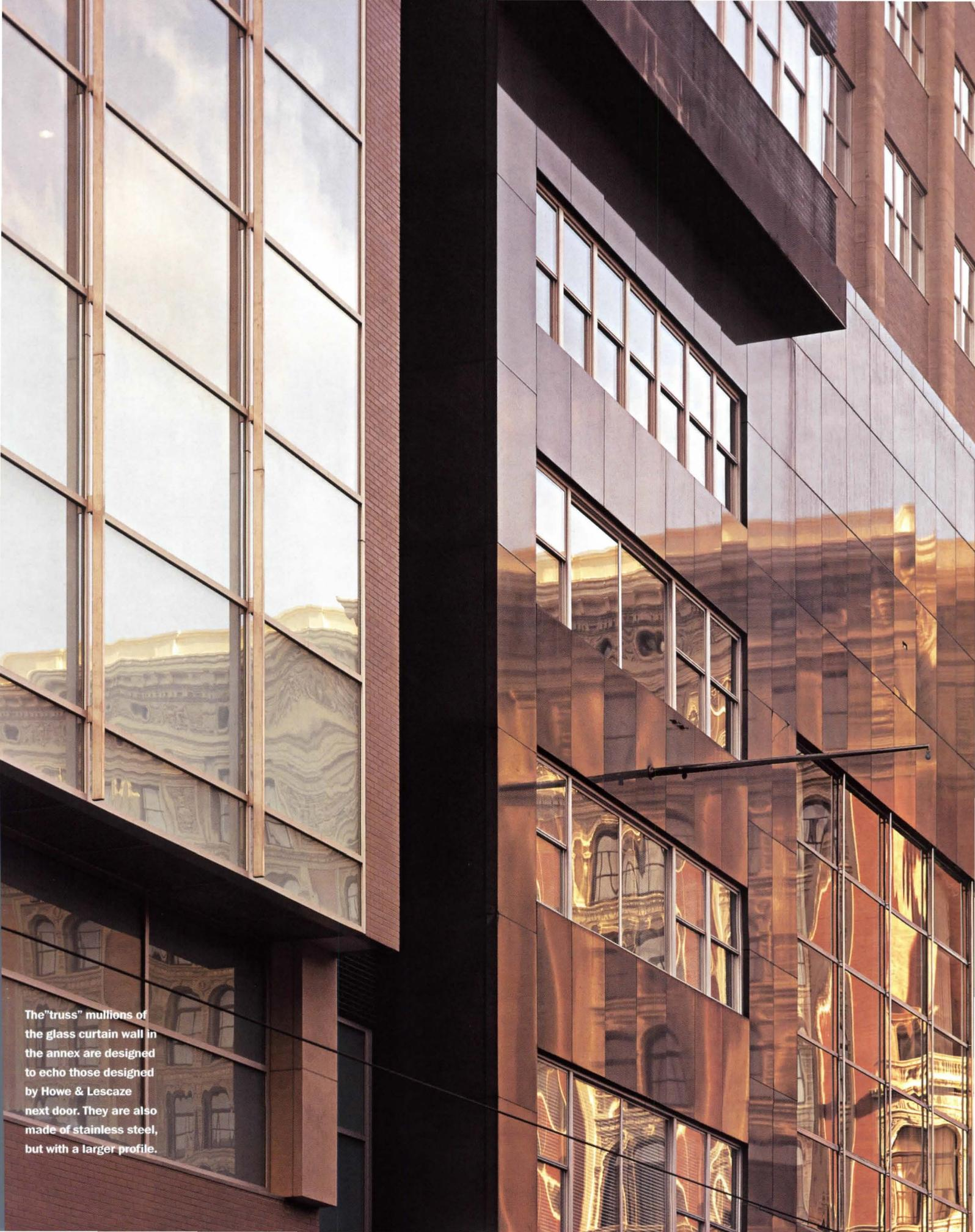
The "truss" mullions of the glass curtain wall in the annex are designed to echo those designed by Howe & Lescaze next door. They are also made of stainless steel, but with a larger profile.
