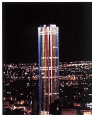
Space Cannon Illumination Inc. introduces the Litehose, the latest in linear lighting technology made of extruded, durable optical-grade acrylic. Available in different diameters and sizes, reflective paints and films are not required. The Focus is an architectural colored luminaire utilizing a 1200w lamp source designed to work with the Litehose or separately. 888-705-1028.
