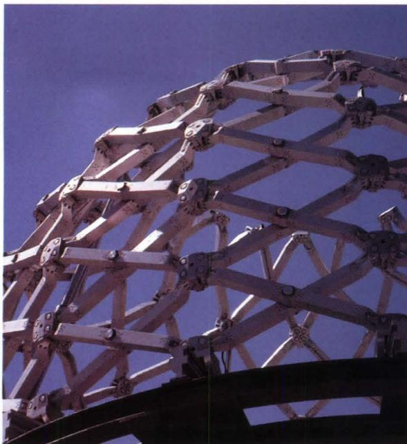
When fully extended, the dome has a height of 15 feet (above). Powered by four digitally controlled hydraulic cylinders, the dome smoothly rises and falls for 18 hours a day.
