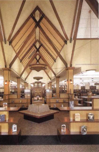
reading room of the Phoenix Central Library, for instance, 30-foot concrete columns support a tensile roof structure, while the location of the room on the top floor allows the monumental space to coexist with standard-height spaces on floors below.
