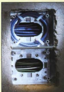
Available in a variety of sizes and configurations, underfloor duct systems provide separate channels for power and data/communications systems. Junction boxes facilitate cable pulling and allow cabling to be added or upgraded. Users access single points of service for workstations through low profile or flush service activations, which may be located anywhere along the duct run.
