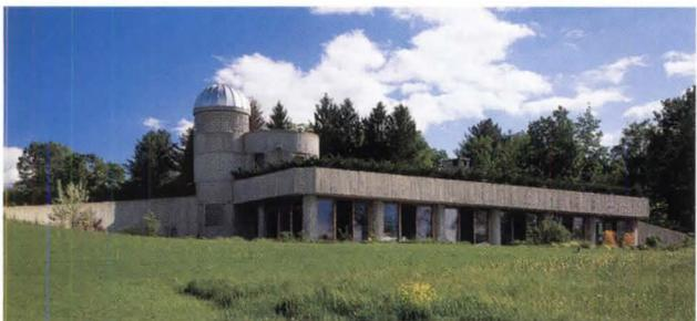
Shrubby takes the place of a railing around the parapet and retaining walls (above and below). Backed by solar panels, clerestory structures sprout from the landscaped roof (top). The silolike form houses a staircase.
