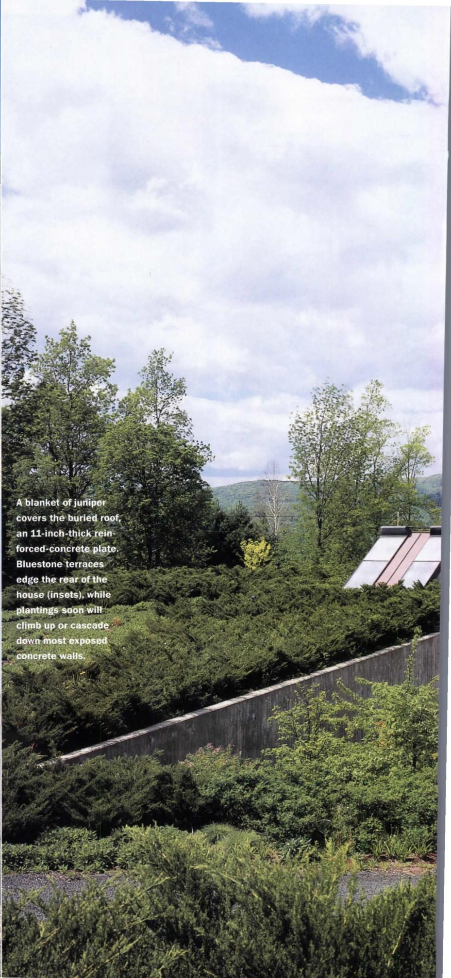
A blanket of juniper covers the buried roof, an 11-inch-thick reinforced-concrete plate. Bluestone terraces edge the rear of the house (insets), while plantings soon will climb up or cascade down most exposed concrete walls.
