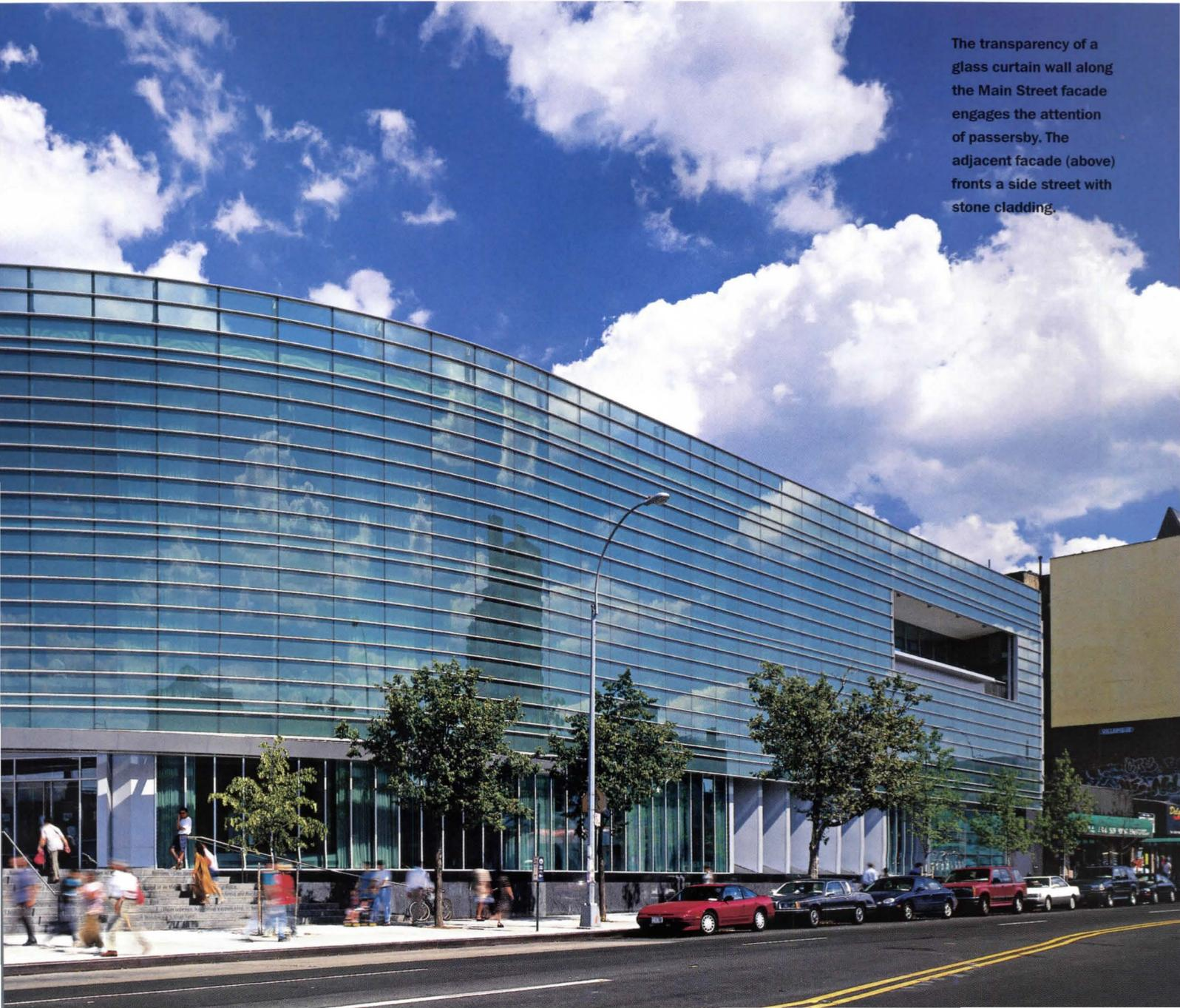
The transparency of a glass curtain wall along the Main Street facade engages the attention of passersby. The adjacent facade (above) fronts a side street with stone cladding.
