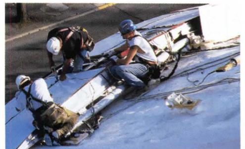
The aluminum pipe girts from which the skin panels hang are connected to steel pedestals. The pedestals, in turn, are anchored to the main
