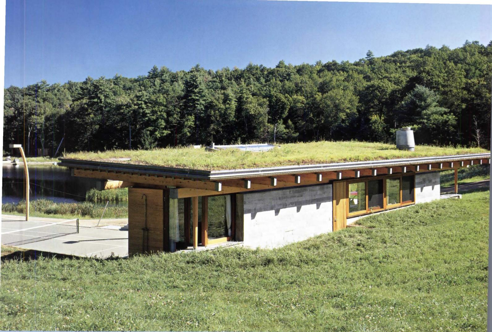
The spruce-framed roof is supported by 10 cypress columns and a wooden box housing the changing rooms
