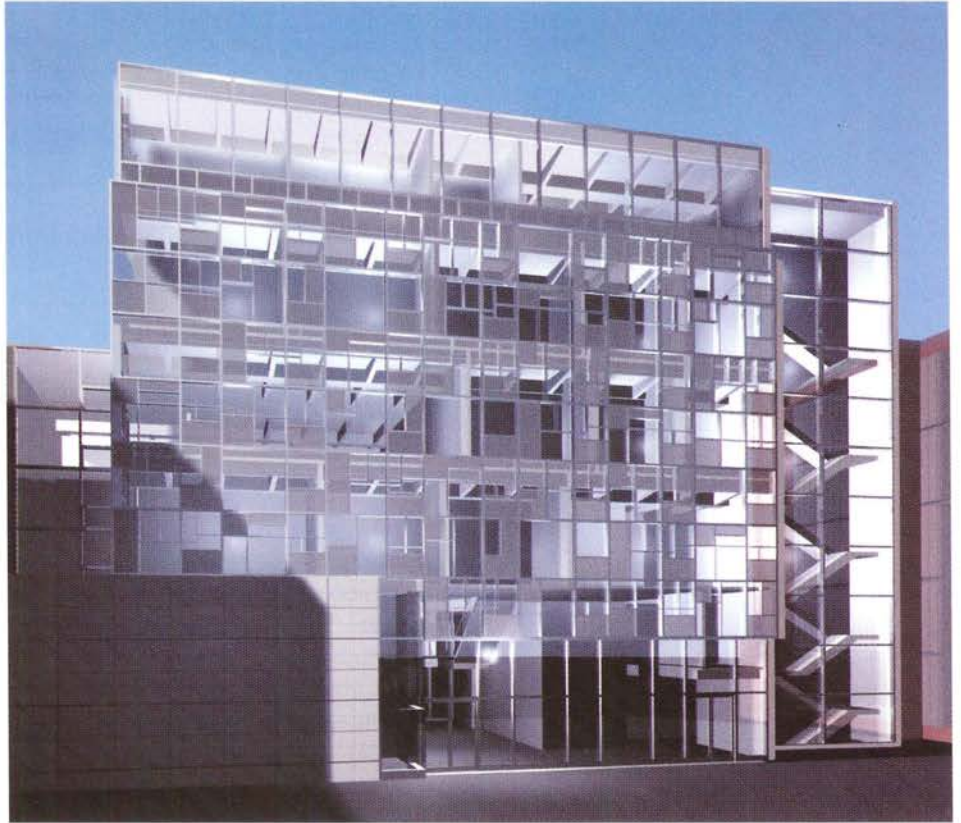
The facade for the Melvin and Claire Levine Hall at the University of Pennsylvania is a factory-made, pressure-equalized, double-glazed unit.
