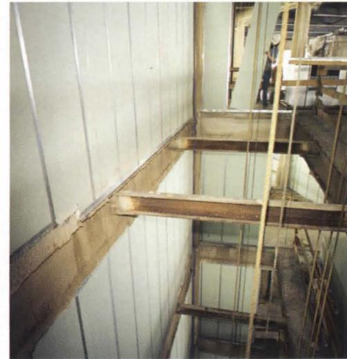
Gypsum shaft walls (seen here from inside the cavity) are the thinnest and lightest-weight shaft walls available.
