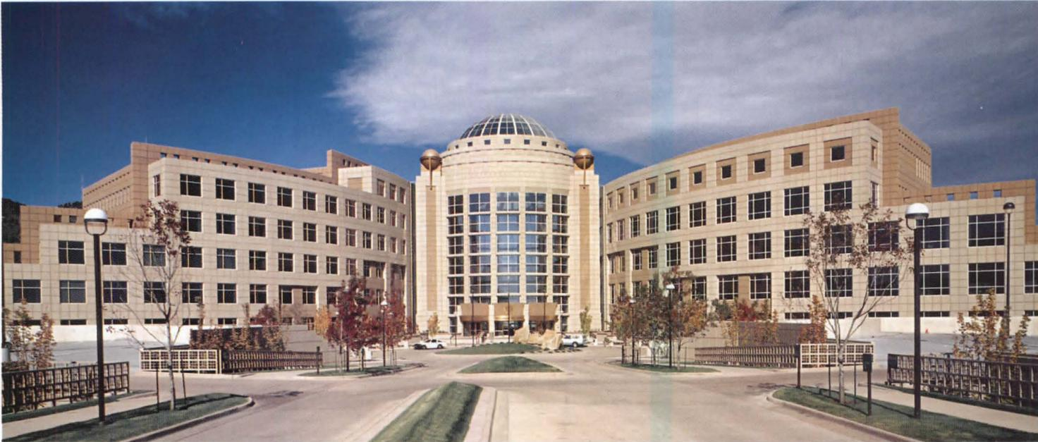
Shape is the major focus of the Jefferson County Justice Center, Golden, Co. More than 400 complex molds with 30 different radii were constructed to produce over 4,000 precast components that form the shell for the structure. Architects: C. W. Fentress and J. H. Bradburn & Associates, Denver
