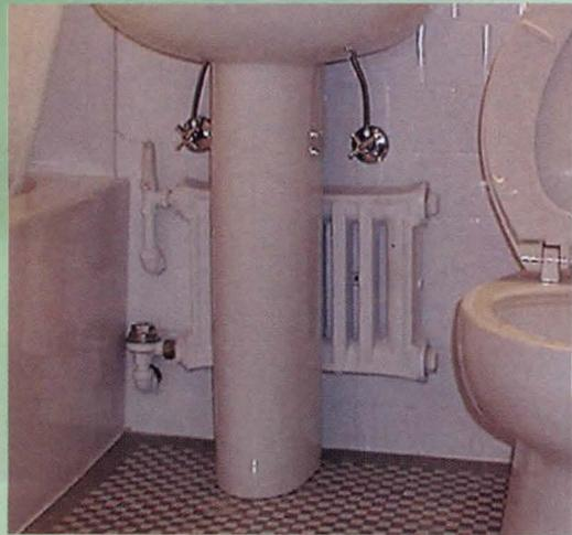
**Before-and-after shots show the effectiveness of blasting the radiators clean with aluminum oxide.**
