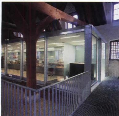
To avoid disturbing archaeological remains in the soil, the new pavilion's foundations are two steel girders that go no deeper than 50 cm. The structure appears to hover above the original floor.
