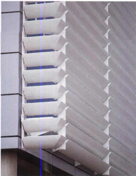
situations. They are manufactured from extruded aluminum sections and may be mounted at a fixed angle or with an adjustable manual or motorized system.
