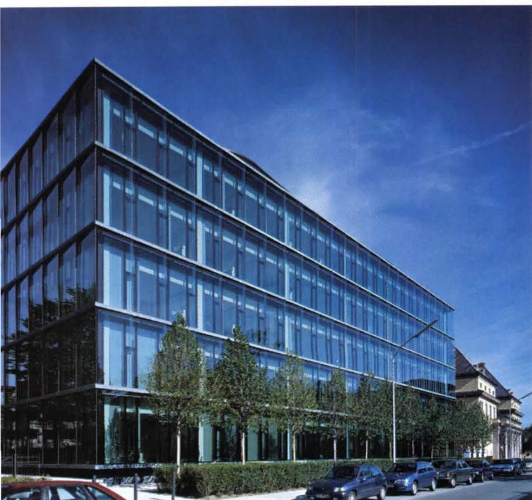
commission by proposing radical cuts and additions to the structure, transforming the monolithic slab into an elongated S-shaped volume that brings interior offices and corridors closer to daylight.
