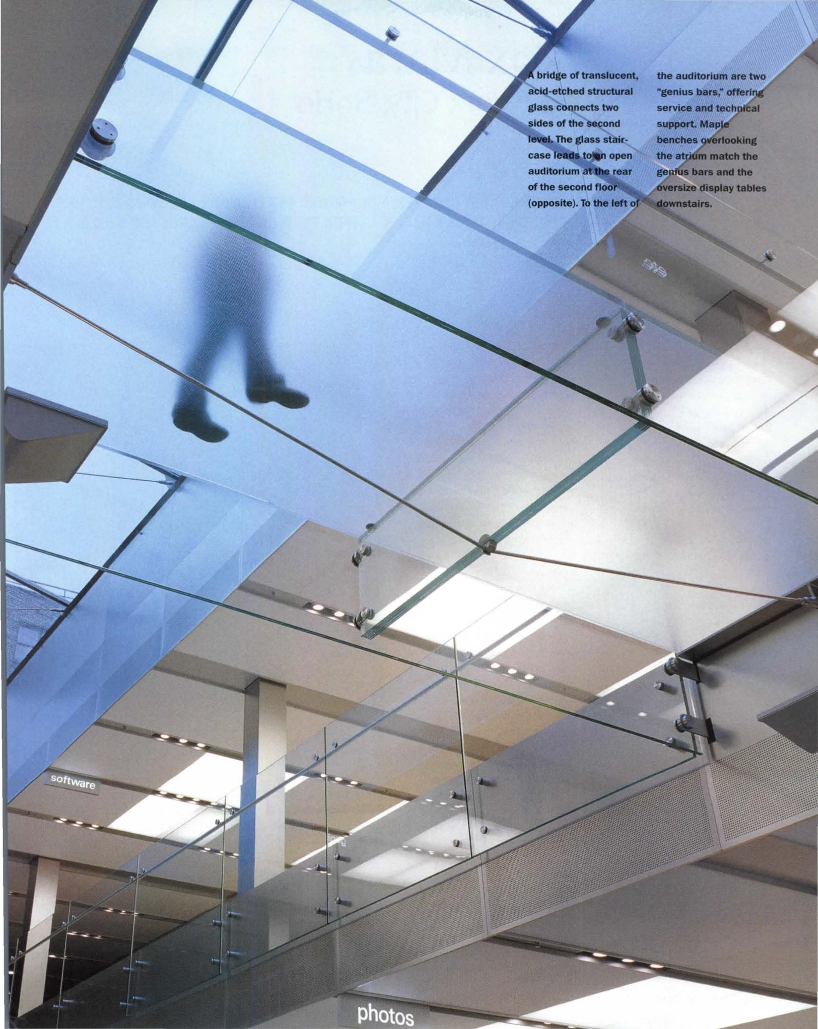
A bridge of translucent, acid-etched structural glass connects two sides of the second level. The glass staircase leads to an open auditorium at the rear of the second floor (opposite). To the left of
