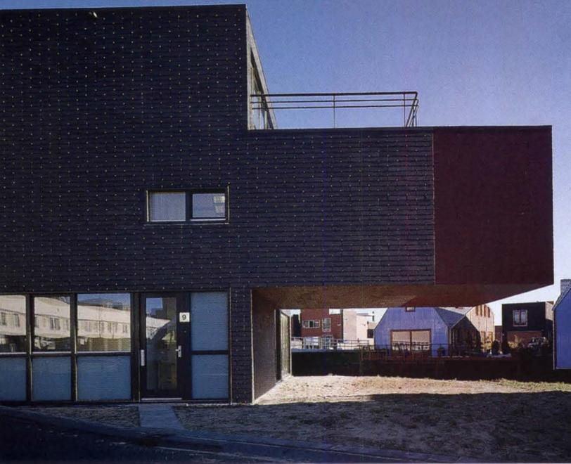
Although all the extensions are fully enclosed, some were originally designed as covered terraces. The architect anticipated that some spaces under the cantilevers might be partly glassed in for sunrooms, but such alterations are not yet permitted.
