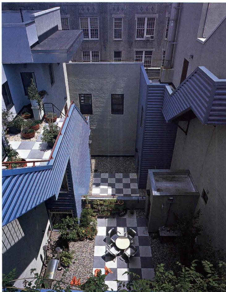
advantage of a zoning regulation that permits mezzanines to be placed in one third of an existing space, and then raised the roofs of the two end buildings by 8 feet, and the middle one by 3 feet. The living rooms of the mezzanine lofts now soar to heights of 16 to 20 feet, while the typical 1,600- to 1,800-square-foot lofts without mezzanines have ceilings that are 9 to 11 feet high.
