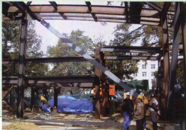
Eric Ko, principal with the project's structural engineer, Arup in San Francisco, noted that time savings are also realized, because unbonded braces can be bolted instead of welded. "Being able to bolt the connections cut 10 weeks off the steel-erection schedule and minimized the need for critical on-site welding," Ko says. Ko also noted that the unbonded braces can be made with circular tube steel that can present an attractive appearance if exposed.
