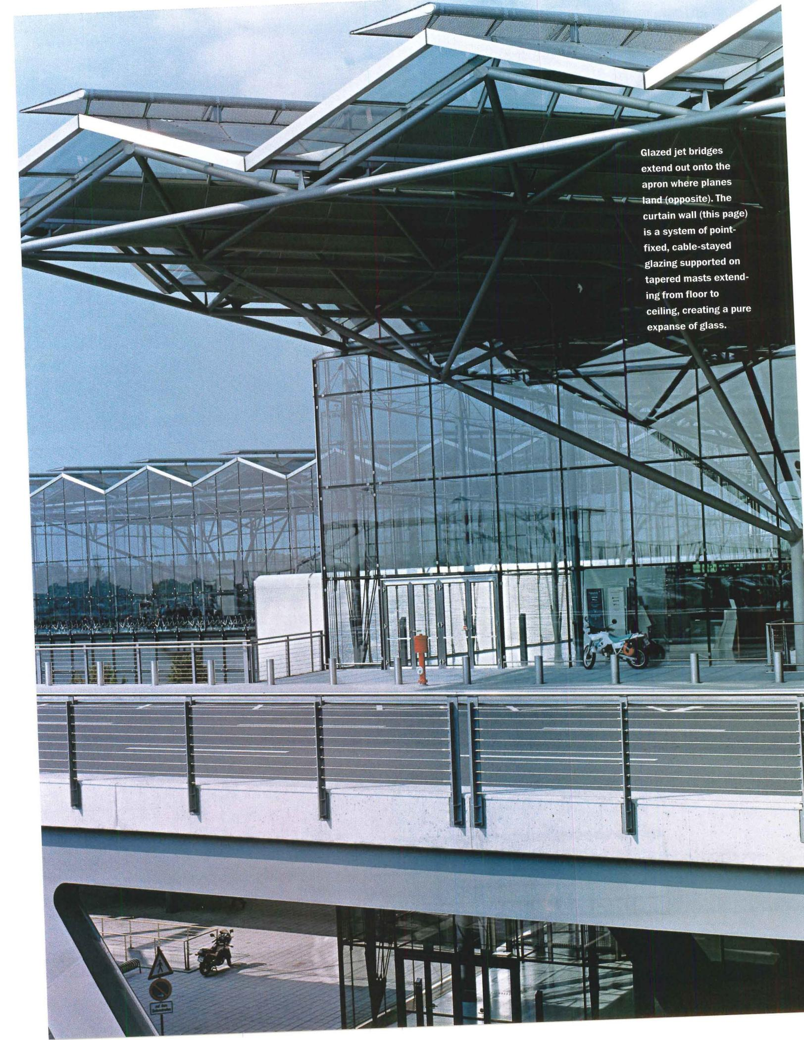
Glazed jet bridges extend out onto the apron where planes land (opposite). The curtain wall (this page) is a system of point-fixed, cable-stayed glazing supported on tapered masts extending from floor to ceiling, creating a pure expanse of glass.
