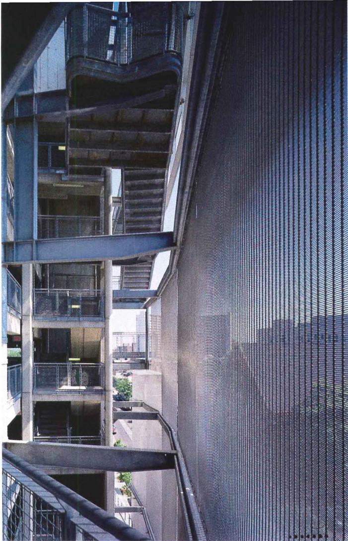
**Stairs and ramps pulled away from the bulk of the 765-car garage work with metal mesh and glass**
