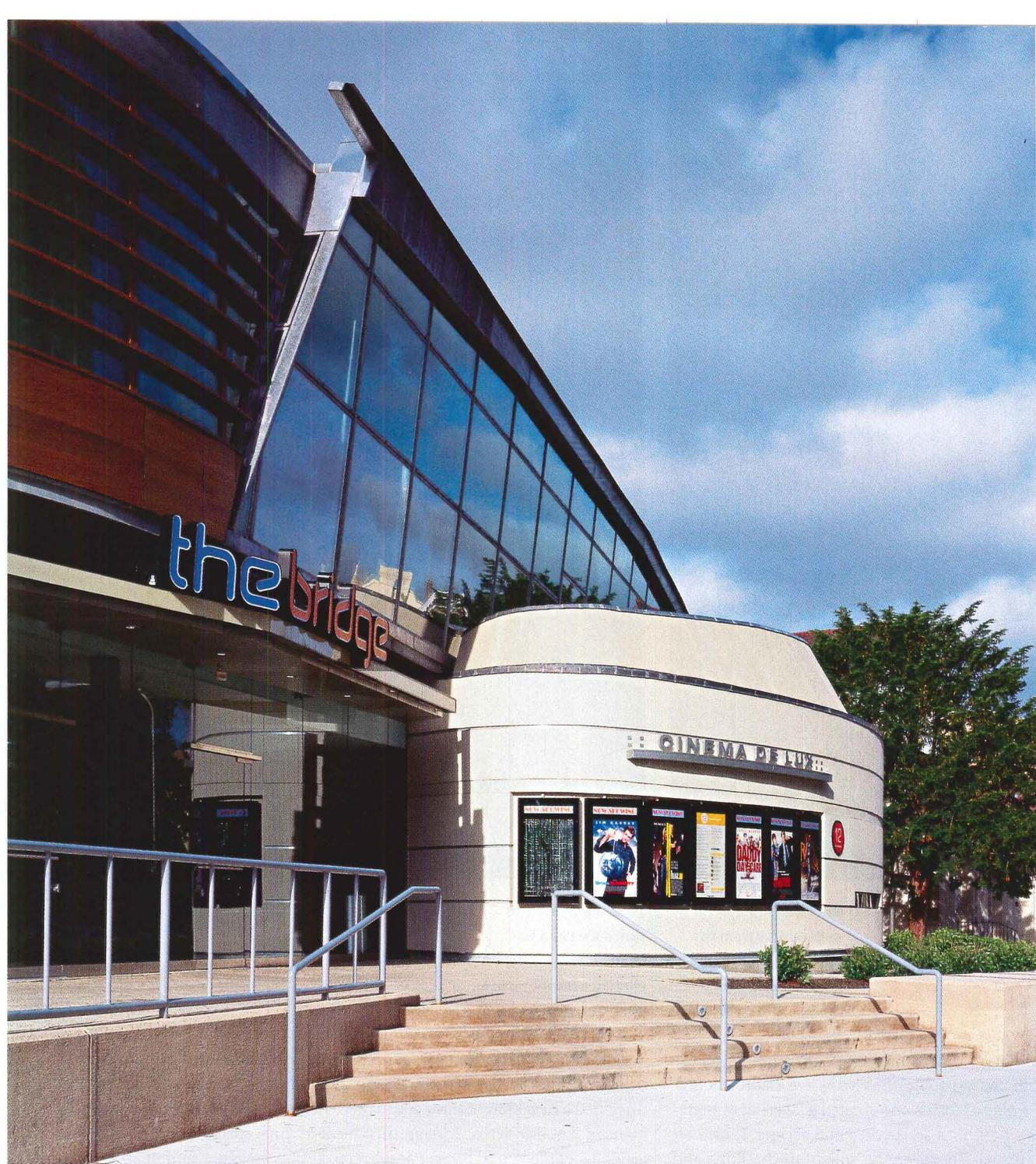
The architects wanted to wrap the curving element protruding from the cinema's main entrance in mahogan and glass, but the tenant used stucco instead (left and opposite). Daylight and outdoor connections are important elements in both the cinema lobby (bottom left) and the café (bottom right).
