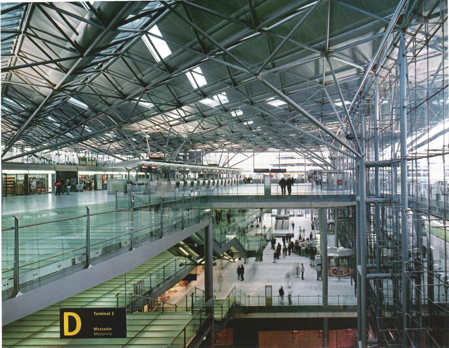
of plate. Terminal Two can be understood as a simple glass shed, or also as a laterally expandable structure, 985 feet long and 246 feet deep, built with prefabricated, modular parts. The physical connection between the two terminals, with which disparate structural systems, is smartly limited to a two-level mass-and-steel bridge.
