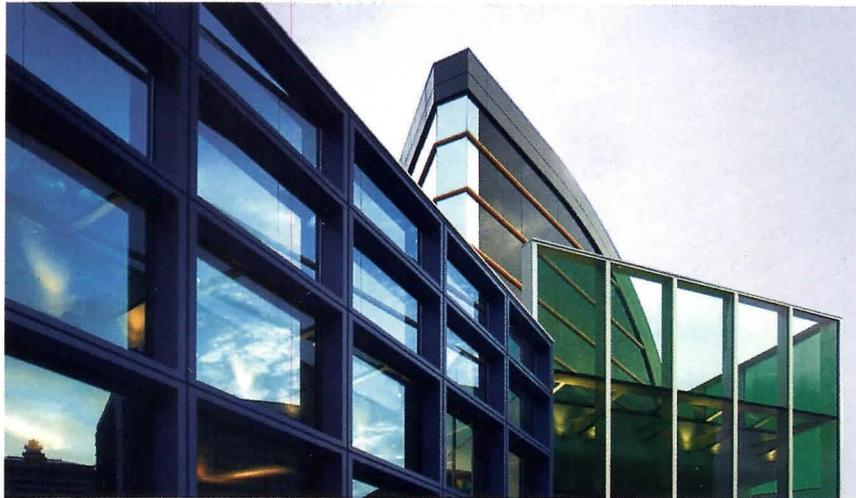
Harmon's contribution involved designing and installing the entire glass exterior addition. (W&W Glass Systems engineered, fabricated, and shipped the system.) This included the "connective tissue" between the newly renovated facility and the newly constructed expansion, plus sloped skylights, a suspended "glass box" entry system, aluminum entry doors, aluminum panels and trim, as well as three different custom curtain-wall systems.
