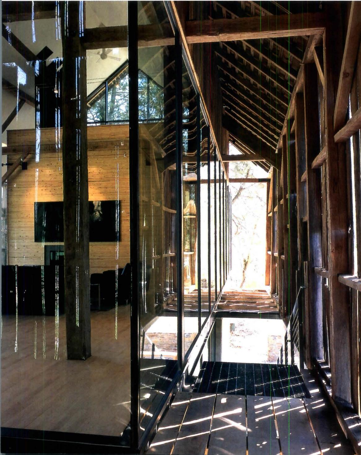
Stock planks, anchored on threaded rods, form the central service core (top row). Part of the barn's original interior has been further enclosed, in glass, while other areas have become more exposed, as in the entry zone where a new steel-grate stair ascends beneath exposed floor joists, arriving in a semi-outdoor porch (left). The glazing accentuates the play of light penetrating slots in the cladding (opposite).
