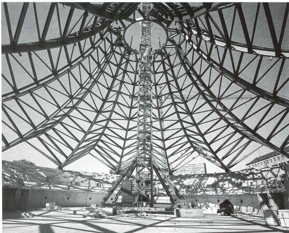
The Tempodrom in Berlin is a folded-steel-plate structure with 5-inch-thick concrete infill panels. A temporary tower was erected to support the frame during construction.
