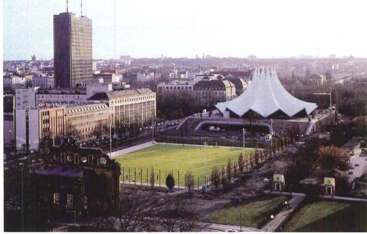
The tentlike form of the Tempodrom is composed of a folded steel-plate structure clad in concrete panels.
