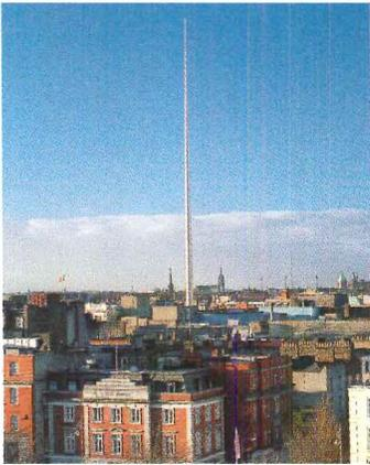
foundries and fabrication shops went into the design, said Robin Cross, the project architect. The spire is built cantilevering into the ground with dampeners to absorb the shock from the structure's movement, which can range up to 3 feet at the apex. The reflective steel is also designed to shift its visual character with subtle changes in daylight and cloud patterns.
