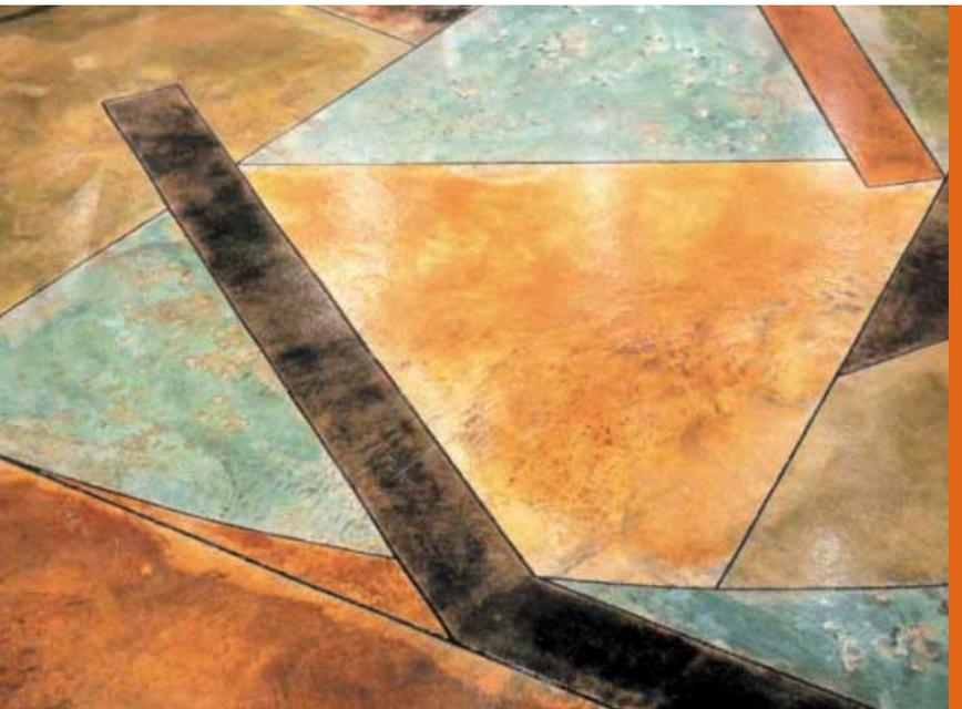
As the durability and cost-effectiveness of concrete make it increasingly popular for interior floors, architects are looking for ways to upgrade its appearance. Chemically reactive stains can be used to color newly cured concrete or to rehabilitate and update existing slabs. Courtesy L. M. Scofield.
