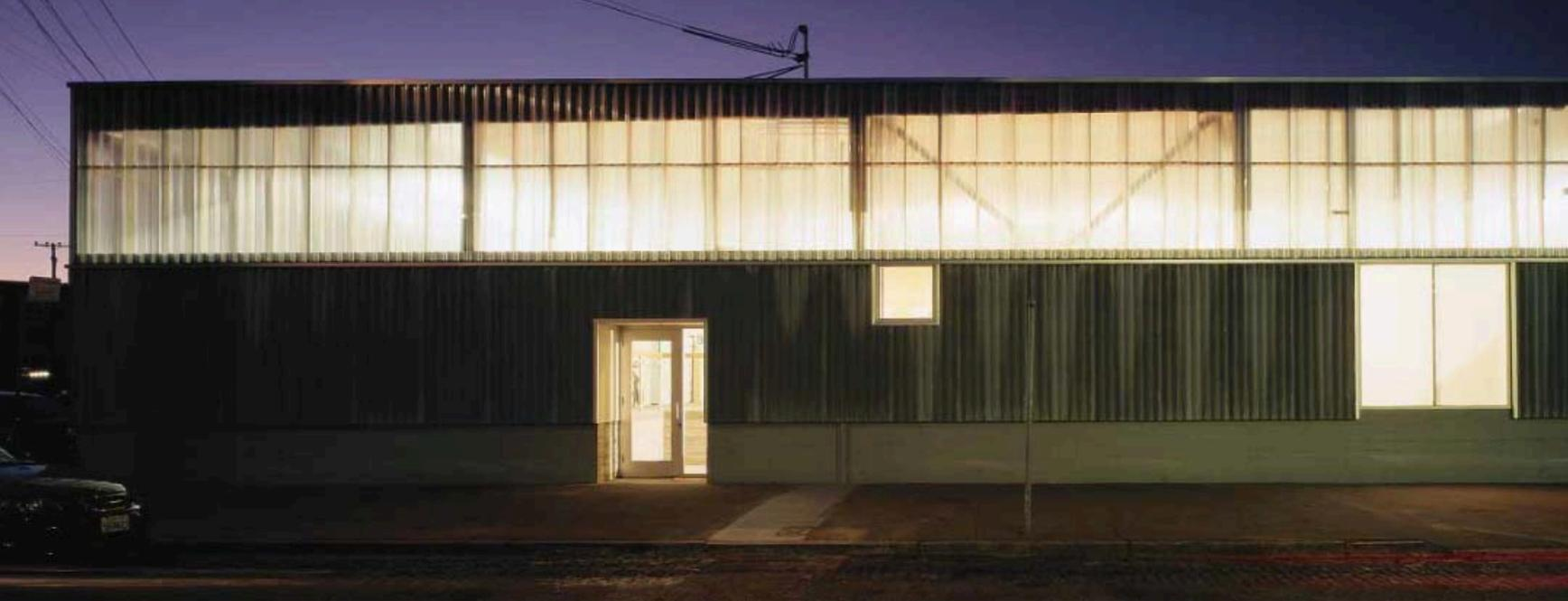
Jensen & Macy wrapped a warehouse in a cement-board base with a polycarbonate clerestory. As light shifts, this simple but skillfully composed and detailed facade changes character, ranging from luminously translucent to opaque (this page and opposite).
