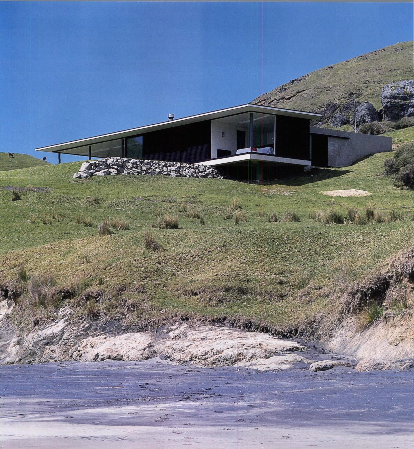
The house is sited along a remote and craggy cove, just where a steep slope levels off into flat, grassy terrain extending out to the surf (above and opposite). The master bedroom, at one corner of the building, cantilevers off the ground. The structure also sits on a low wall of stones, collected from the site (above).
