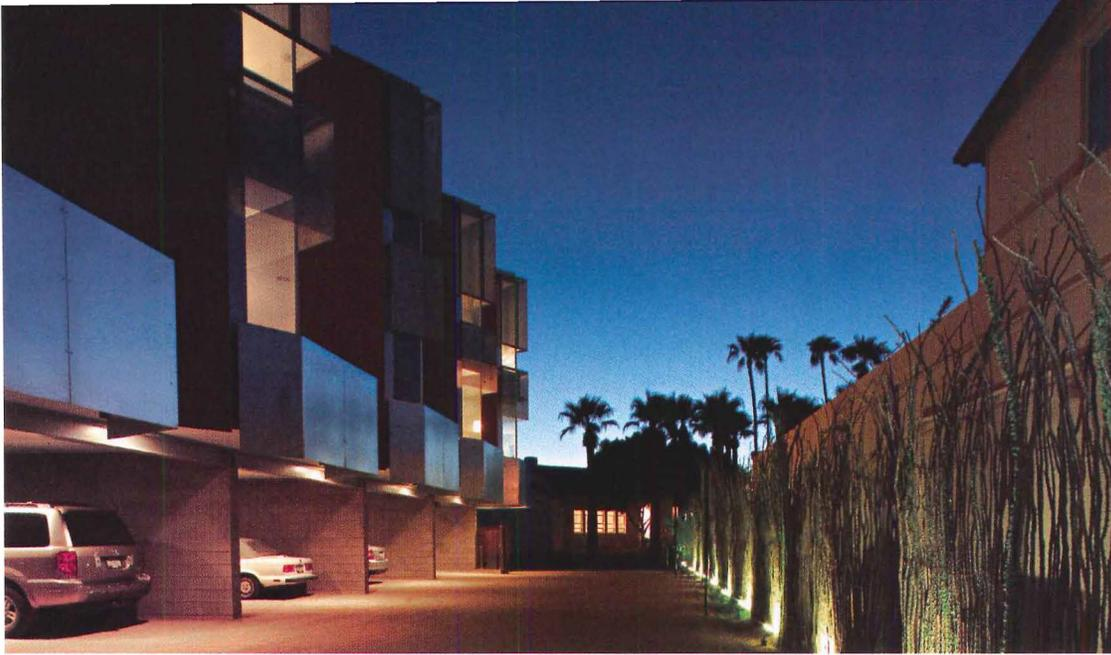
Bruder used his most expensive material—zinc—on the building's street front and accented it with vertical slots of glass (below). Balconies turn to capture views of the mountains and are shaded by perforated-metal veils (left).
