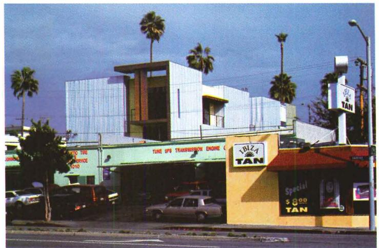
conies in the front—one completely open, the other shielded by rusted-steel louvers—create a physical and psychological relationship to the street. A steel window box offers an unobstructed view of the private life within.
