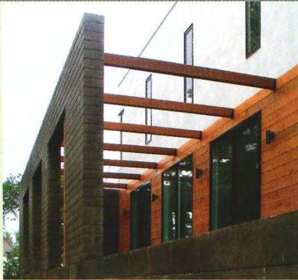
ing space, and a concrete veneer wall that transforms into a freestanding garden wall. A large second-floor window with an overhead garden trellis offers framed views of the neighborhood.
