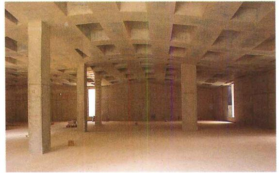
Each stele was lowered into place with a crane (left). Formwork for the coffered ceiling (middle) followed the site's lines, and the concrete was left uncoated (right).
