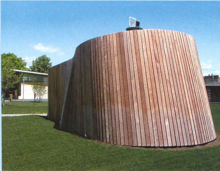
“The bid set for the camera obscura focuses on the process of making rather than just describing,” explains SHoP partner William Sharples. With construction simulated on the architect’s computers, bidders were offered pictorial schedules of beams and connectors in 3D, similar to drawings in a toy model kit.
