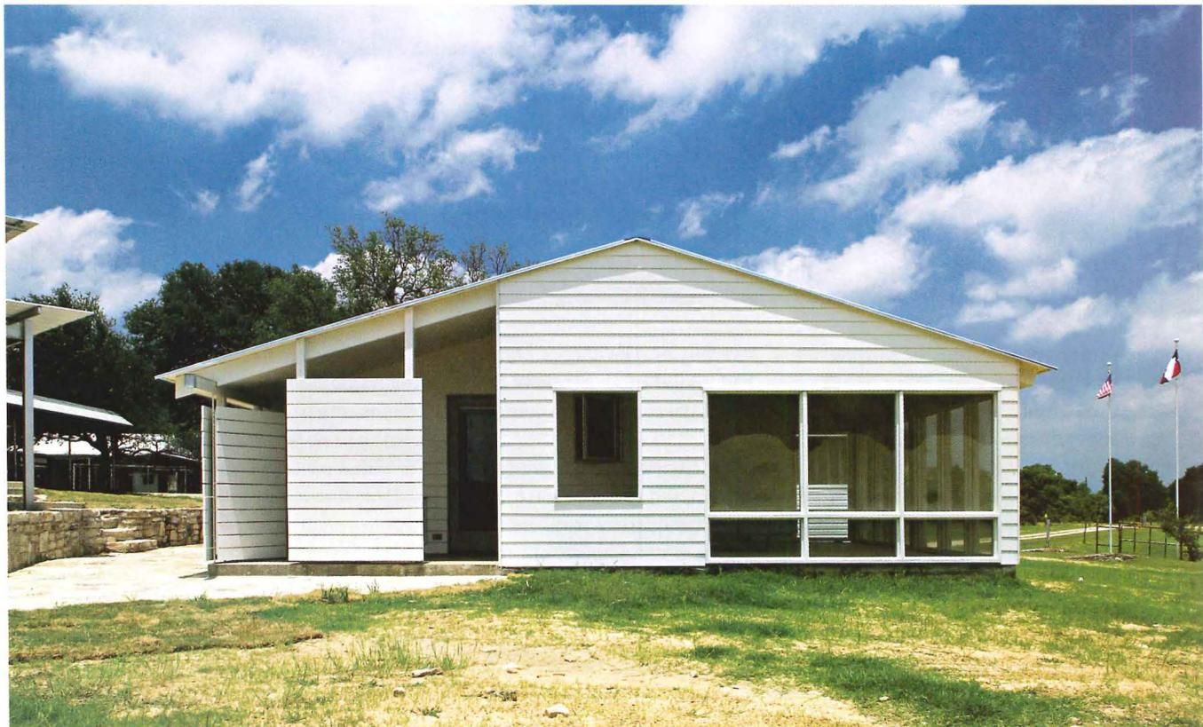
The architect layered corrugated plastic against perforated metal sheets on the lower half of the walls, allowing diffused natural light into the space
