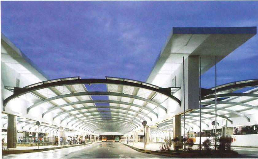
The roof of Nucleo de Arquitetura's Lapa Bus Terminal expels exhaust while filtering sun.
