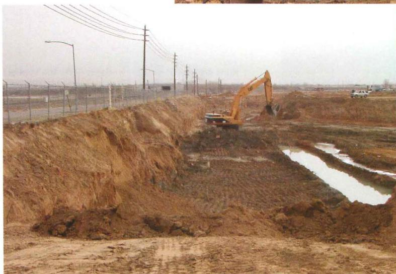
Parsons' contractors scraped nearly 5 million tons of soil, both contaminated and clean, from the surface of the abandoned Stapleton International Airport. In some areas, contractors dug down as far as 25 feet. Once the 3-to-5-foot-deep "smear zone"
