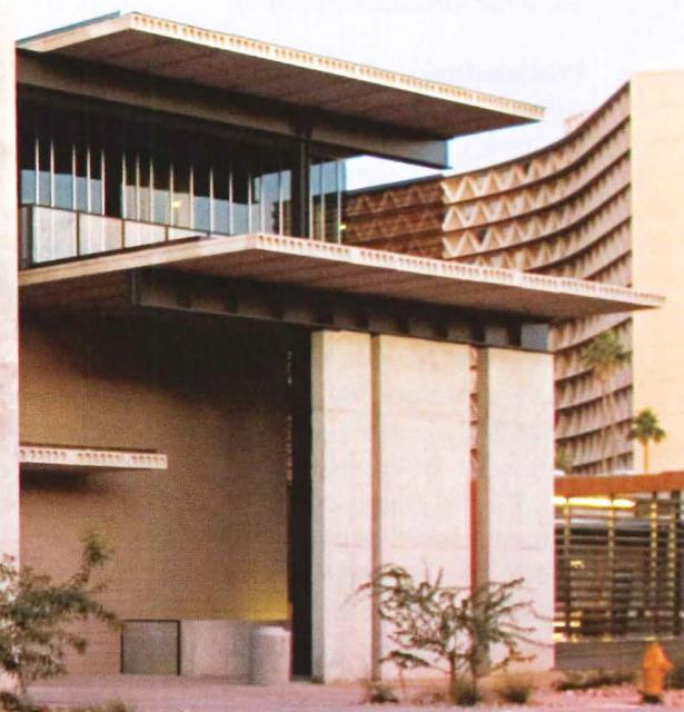
trusses, the height of one floor, dampen vibrations for the heavy-duty activities in the labs and, between the two floors, carry a mezzanine on their lower chords to accommodate smaller labs and walkways (section, opposite).
