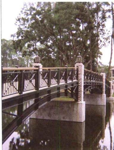
New and improved architectural styles and looks are often custom designed to provide superior aesthetic appeal. One such new approach is the "Archway" Style Bridge, a new pedestrian and vehicular truss style from Steadfast Bridges. The Archway differs from other Steadfast Bridge styles in that it features a cambered bottom chord that emphasizes a traditional arched design. This allows for open clearance above the bridge deck while enhancing the aesthetic beauty and distinction below the deck.
