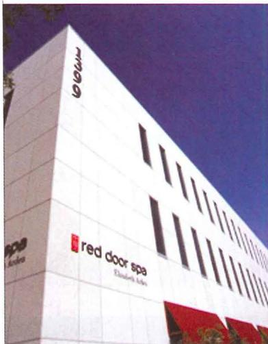
Thin lightweight natural stone wall cladding by THIN STONE SYSTEMS, LLC offers economical solutions for new construction and renovation, for both exterior and interior. Reinforced by a special patented process, the thin veneer panels of natural granite, marble, or limestone are applied to a structural framing system of extruded aluminum. Weighing only 6-lb. psf, the wall system provides many advantages including speed and simplicity of installation.
